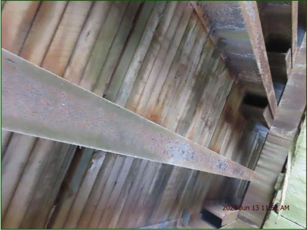
Description: Curbs: Light weathering and light rot throughout.
