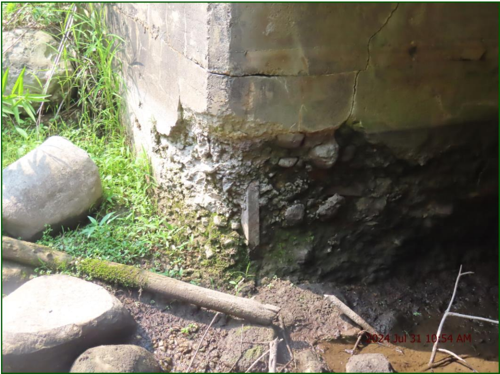
Description: Inlet: Severe spalling and disintegration.
