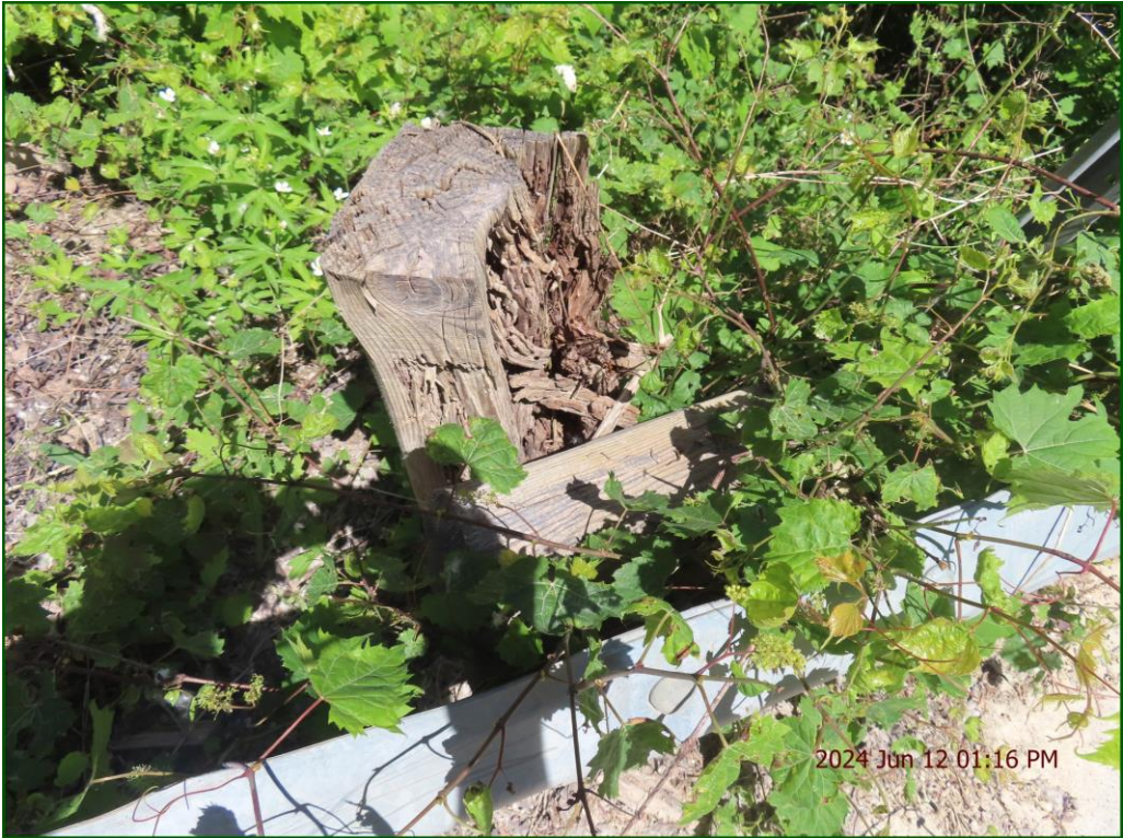
Description: Railing systems: Severe rot.
