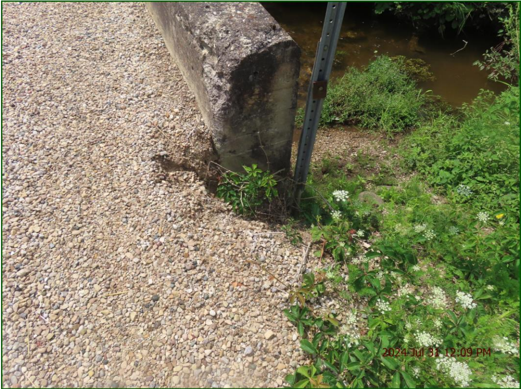
Description: Embankments: Minor erosion on north-east quadrant.
