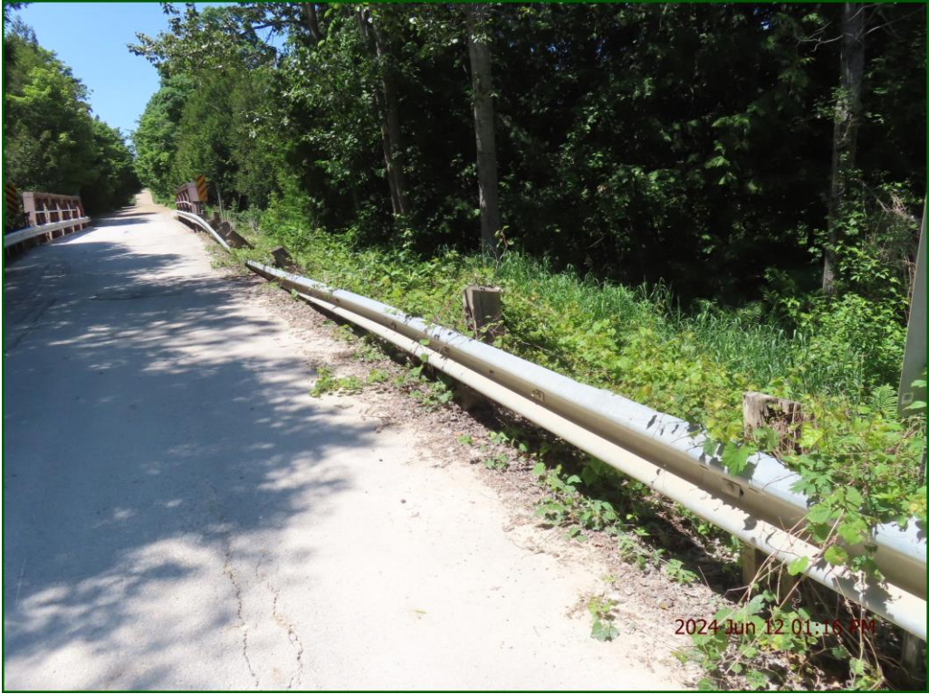
Description: Railing systems: Severe rot.
