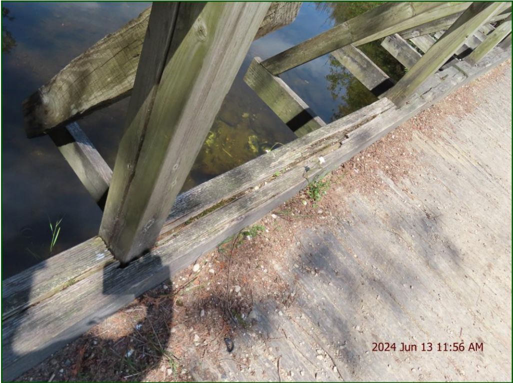
Description: Curbs: Light weathering and light rot throughout.
