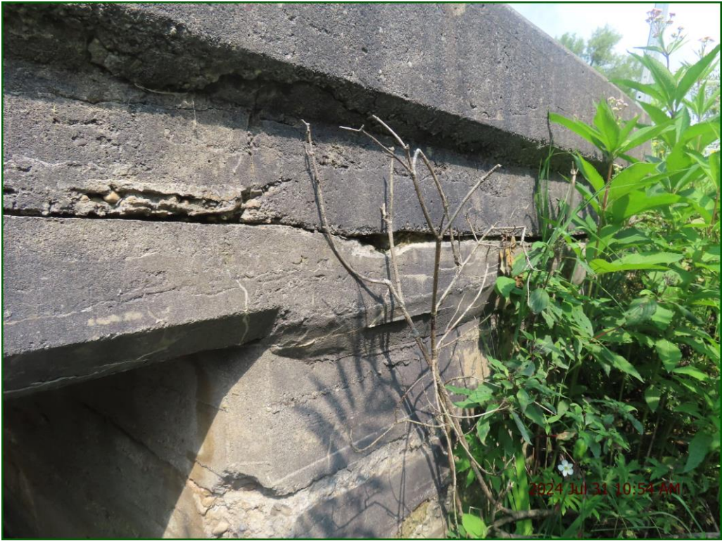
Description: Inlet: Severe spalling and disintegration.
