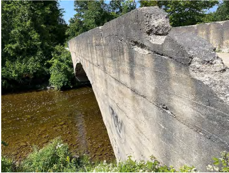
Figure 25: The North Line Saugeen River Bridge (A.S.I., 2023).
