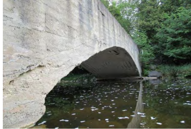
View of Structure Elevation
