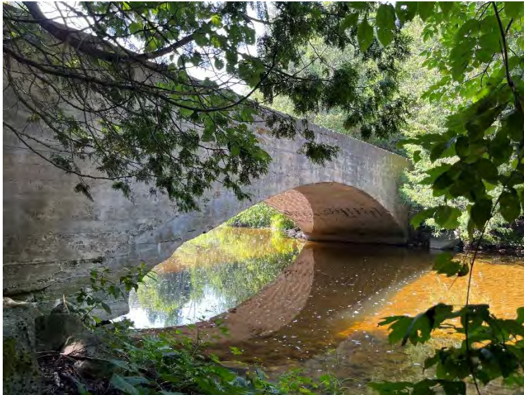
Plate 1: North elevation of Northline Road Culvert, looking southwest (A.S.I., 2023).
