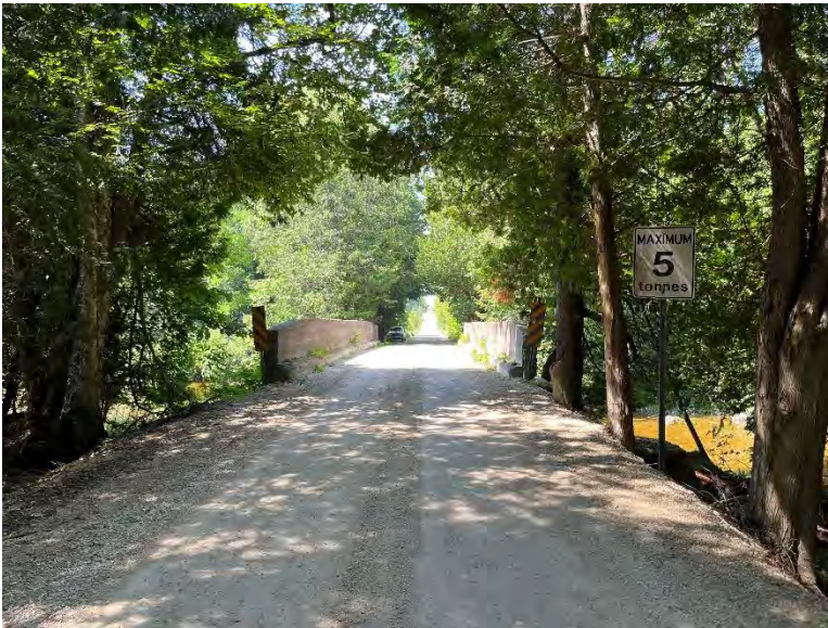
Figure 12: Eastern approach to the Northline Road Culvert, looking west (A.S.I., 2023).
