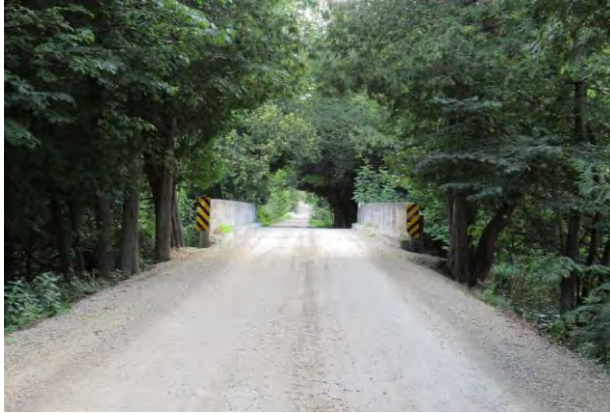
View of Structure from West Approach
