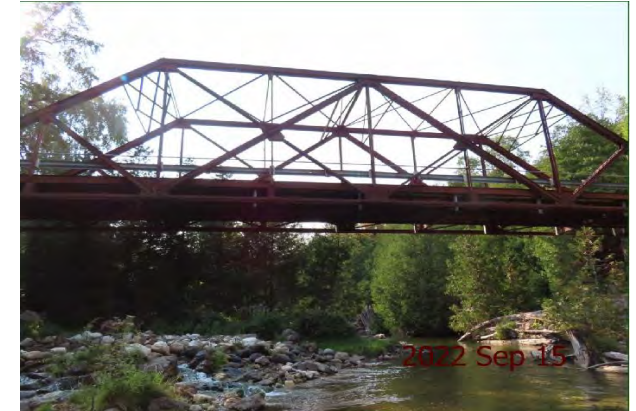
View of Watercourse Downstream
