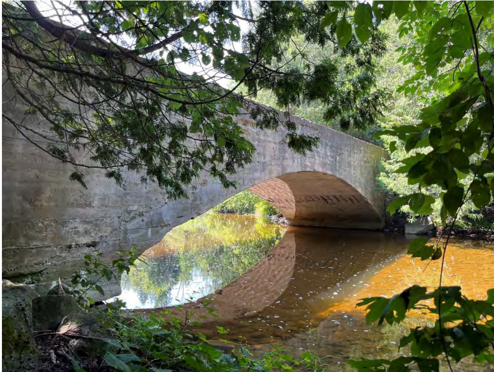
Figure 2: South elevation of the Northline Road Culvert (Structure 44), looking northeast (A.S.I., 2023).
