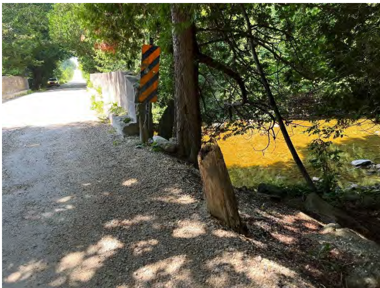
Figure 20: Trees and tree stumps right next to the culvert's northeastern abutment (A.S.I., 2023).
