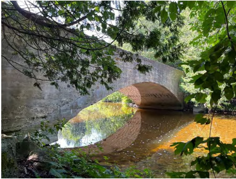
Figure 9: North elevation of Northline Road Culvert, looking southwest (A.S.I., 2023).
