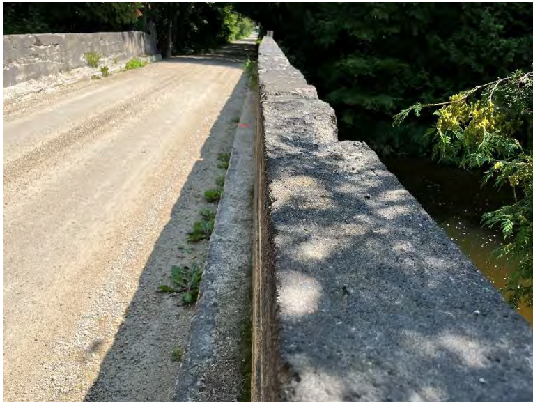
Figure 16: Detail view of southern concrete barrier (A.S.I., 2023).
