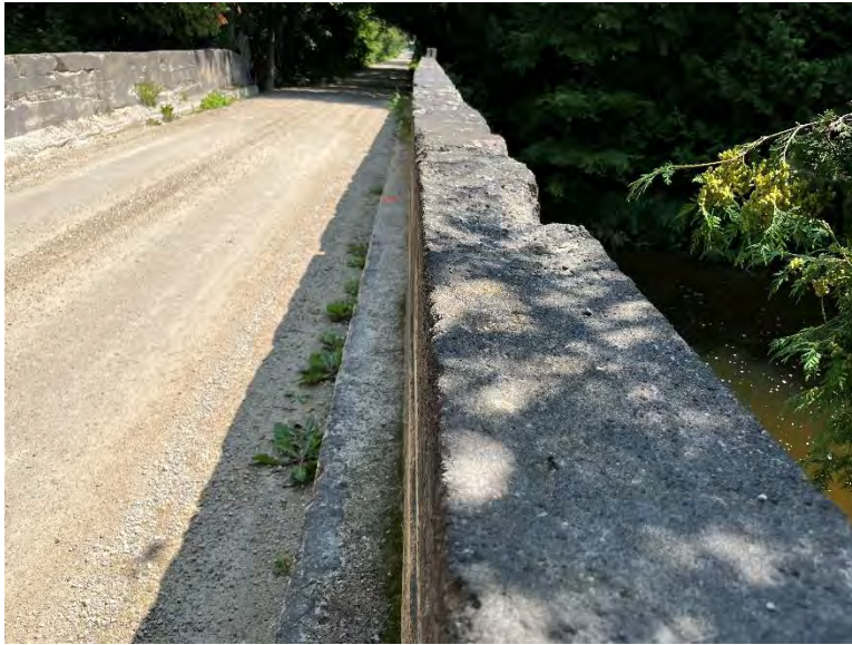
Plate 8: Detail view of southern concrete barrier (A.S.I., 2023).
