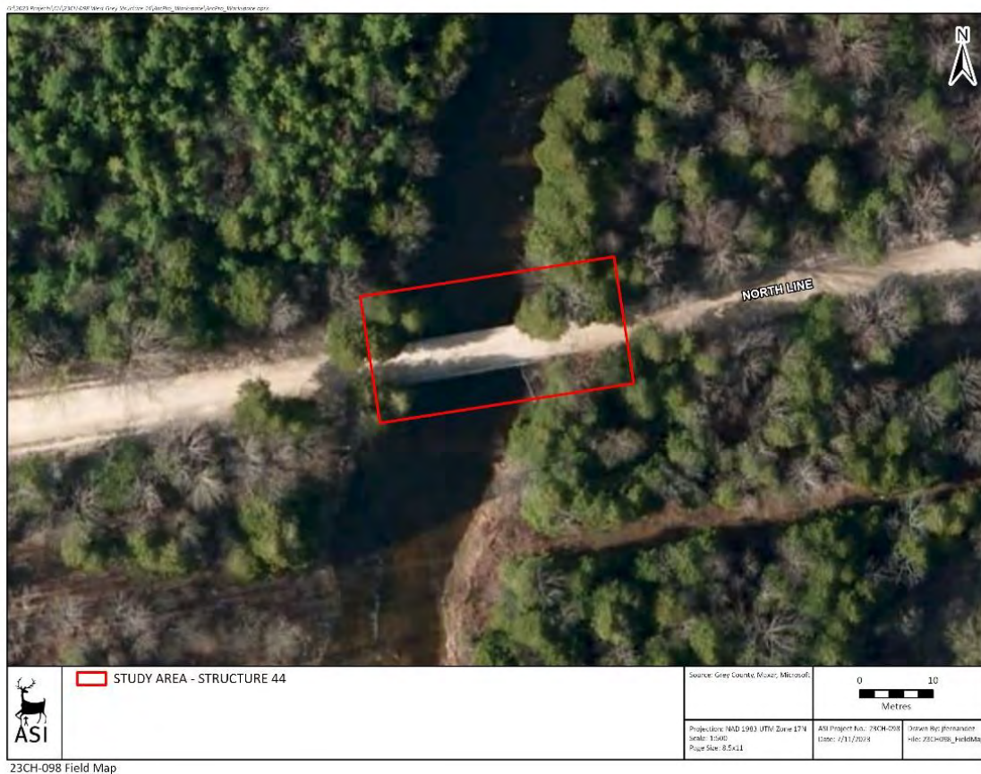
Figure 3: Aerial image of the subject bridge in the Municipality of West Grey (Google Maps)
