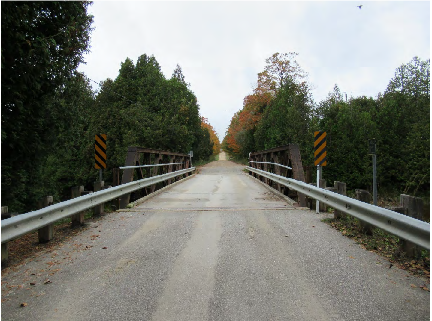
Image 8 – G-040 View from East Approach
