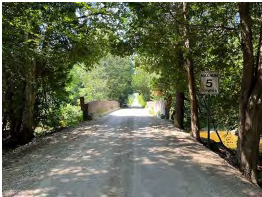
Image 6: Northline Road Structure 44; roadbed disturbed, no archaeological potential.
