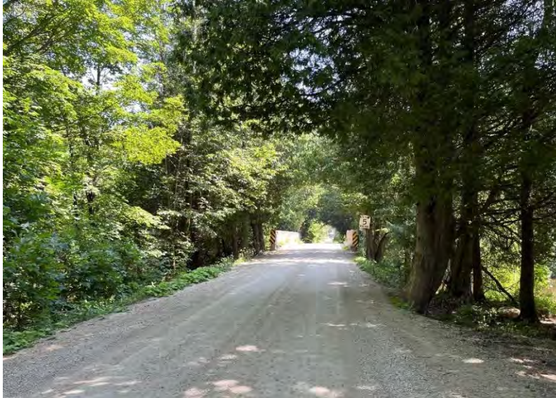
Image 1: Northline Road Structure 44; test pit survey required beyond disturbed gravel roadbed.
