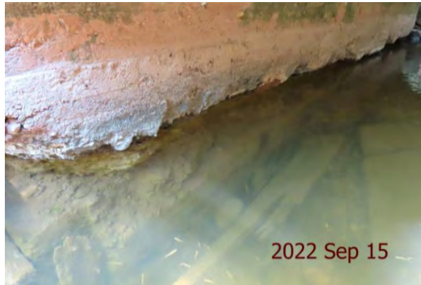
Barrel: Severe scouring and disintegration at waterline
