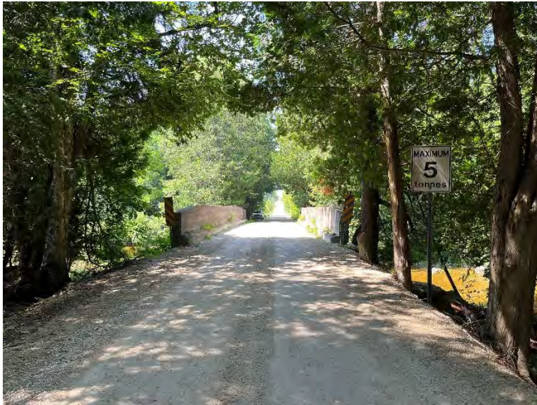
Plate 4: Eastern approach to the Northline Road Culvert, looking west (A.S.I., 2023).
