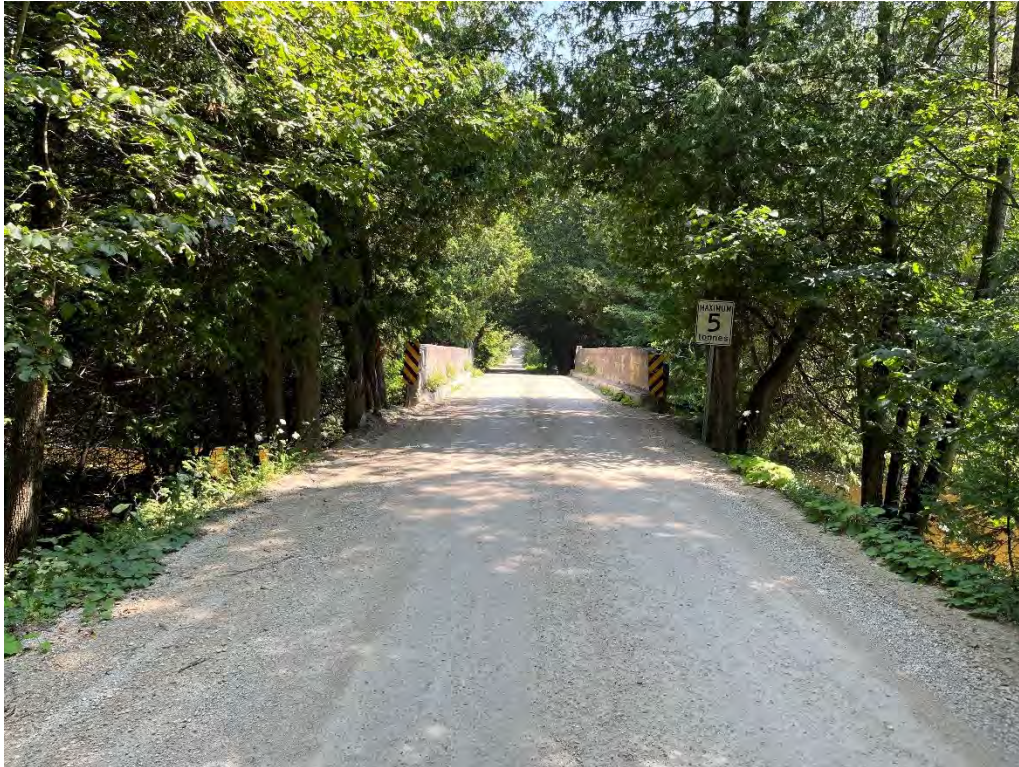
Figure 23: View of the Northline Road Culvert and surrounding wooded area, looking east (A.S.I., 2023).
