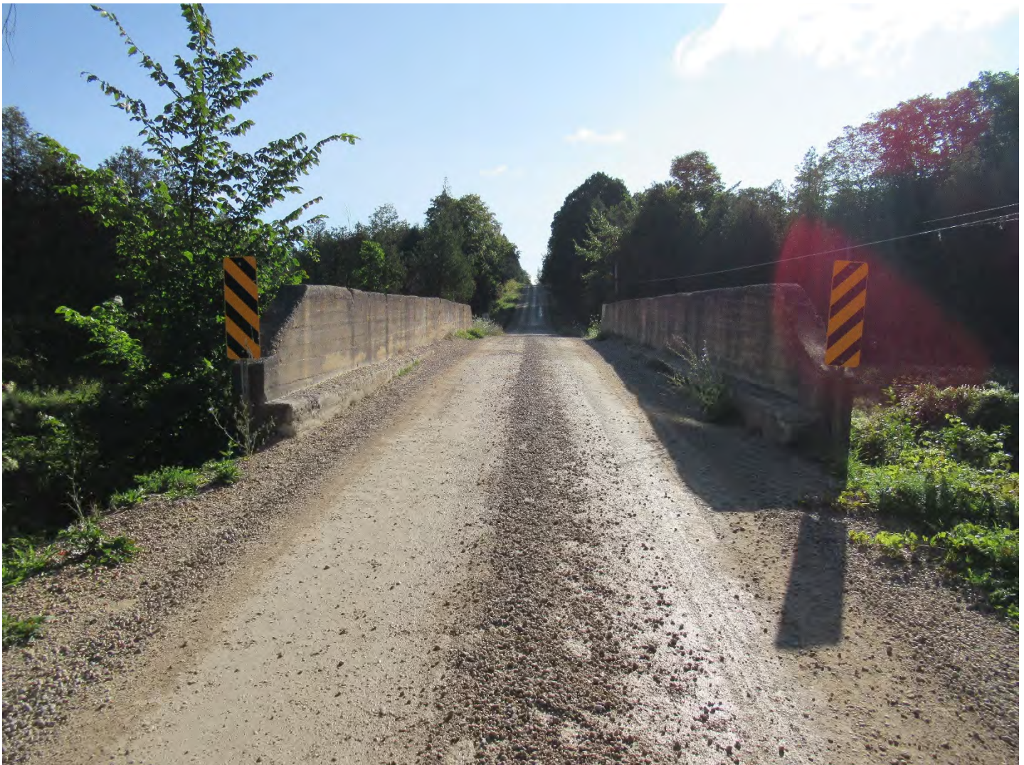
Image 6 – G-038 View from East Approach
