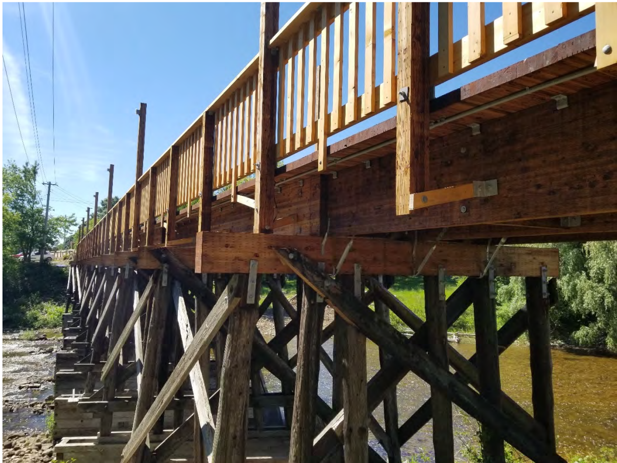
Image 12 – P-101, Durham Pedestrian Bridge Elevation View
