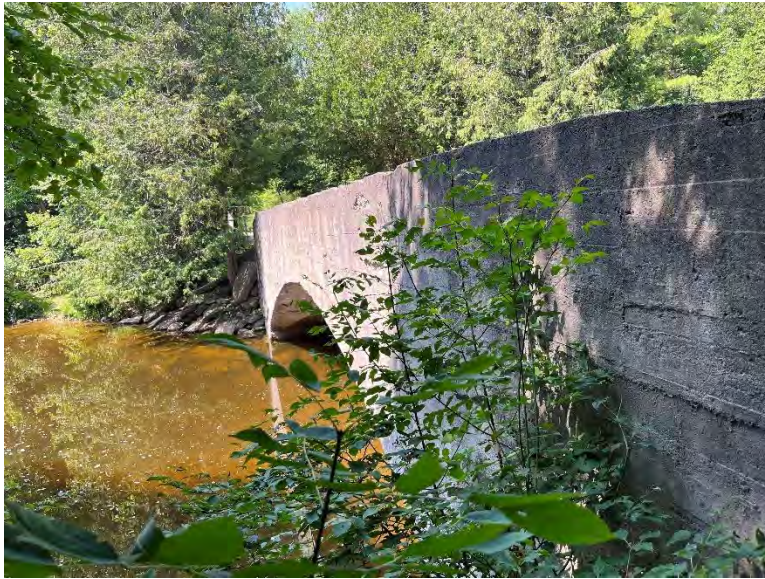
Plate 2: South elevation of the Northline Road Culvert, looking west (A.S.I., 2023).
