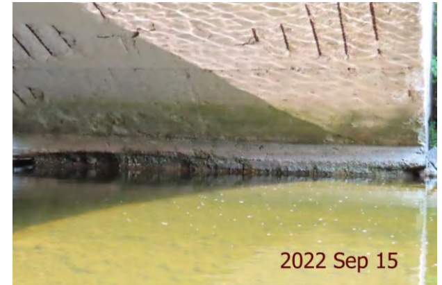
Barrel: Severe scouring and disintegration at waterline
