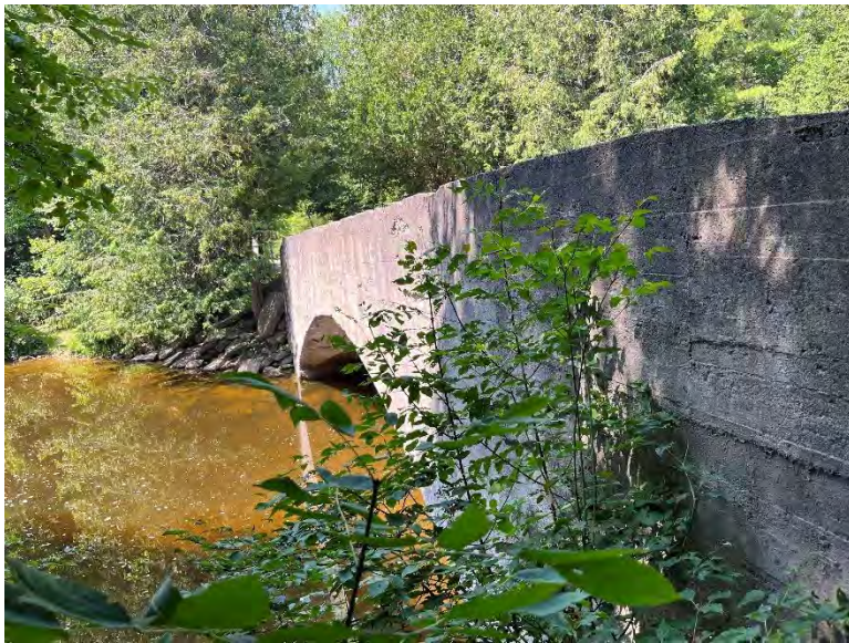
Figure 10: South elevation of the Northline Road Culvert, looking west (A.S.I., 2023).
