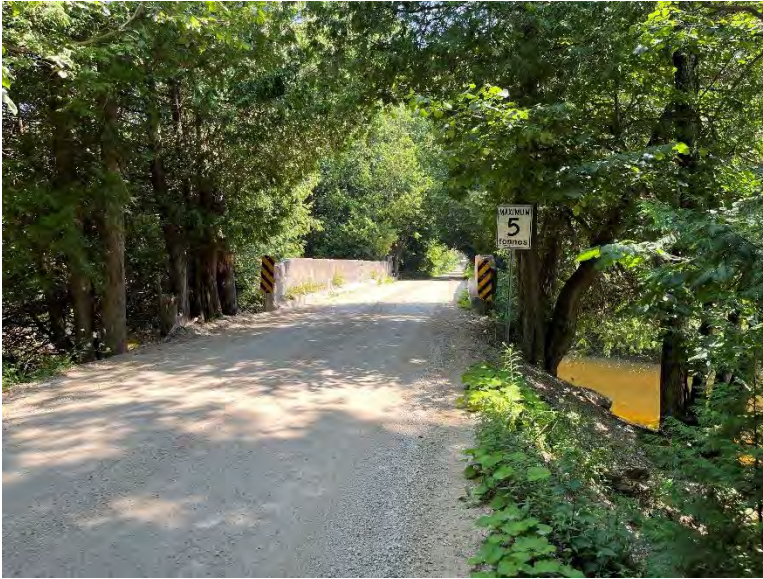
Figure 11: Western approach to the Northline Road Culvert, looking east (A.S.I., 2023).
