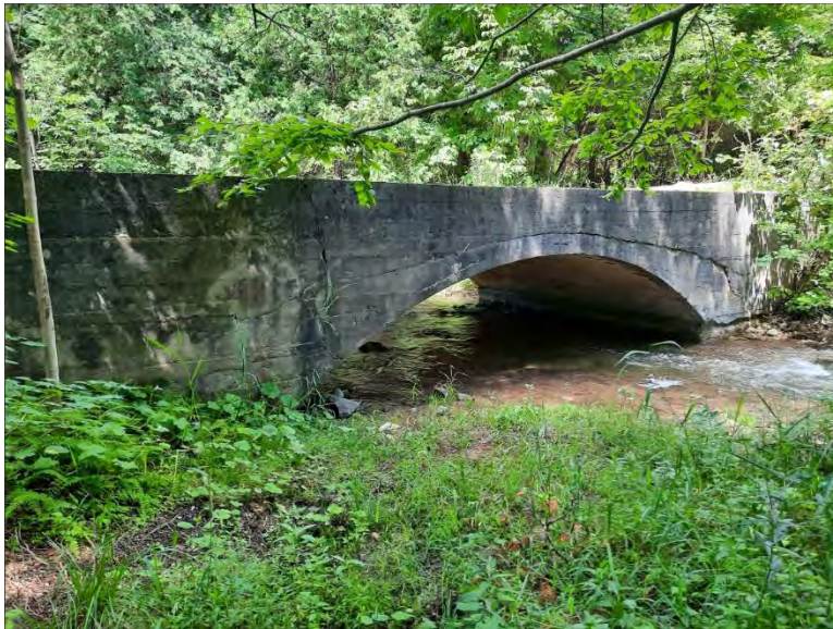
Figure 24: One of the Twin Bridges ( historicbridges.org ).
