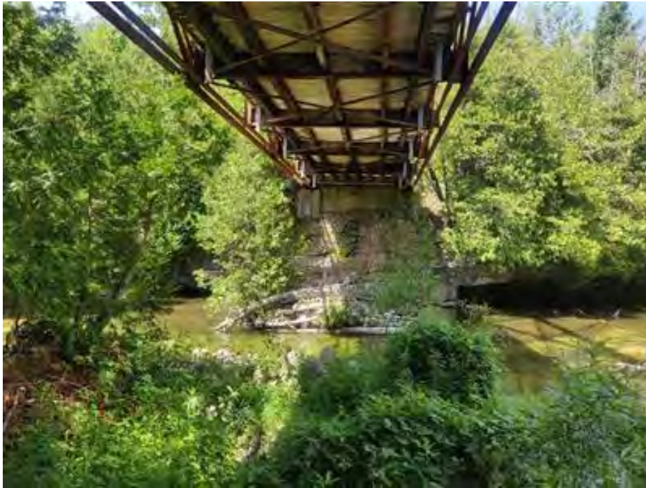
Image 11: Traverston Road Structure 33; stabilized bank disturbed, no archaeological potential.
