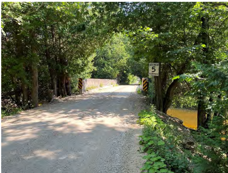
Plate 3: Western approach to the Northline Road Culvert, looking east (A.S.I., 2023).
