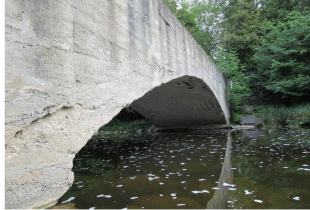
View of Structure Elevation
