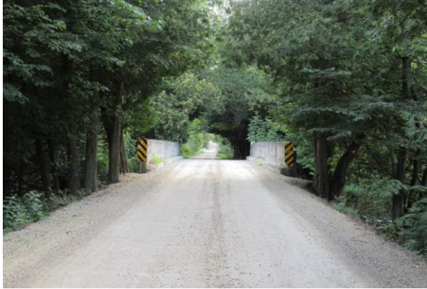
View of Structure from West Approach
