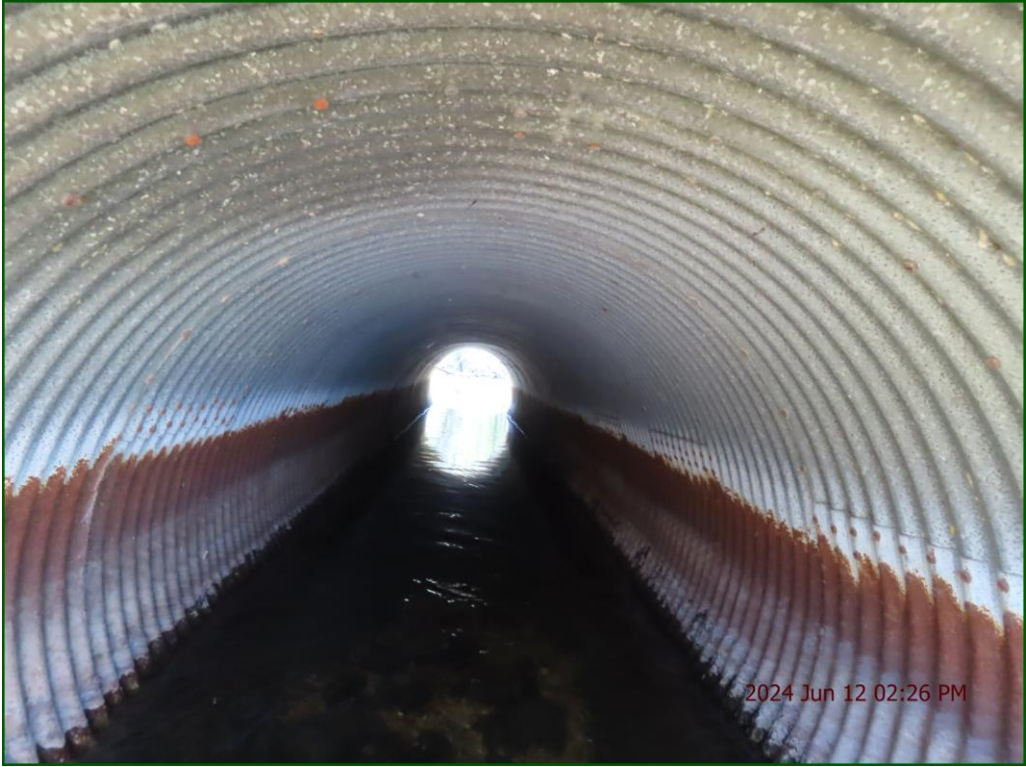
Description: Barrel: Separation of sections at mid point of south barrel.
