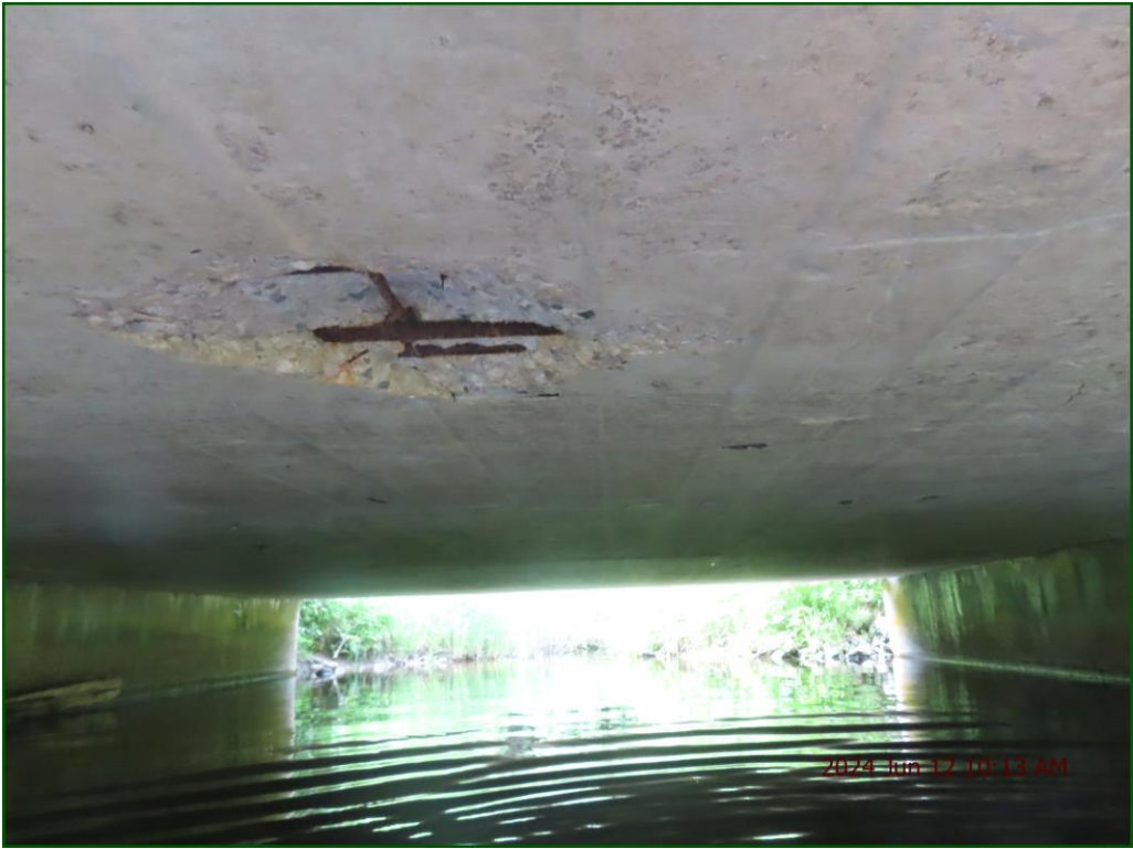
Description: Barrel: Severe localized spall with exposed reinforcing.
