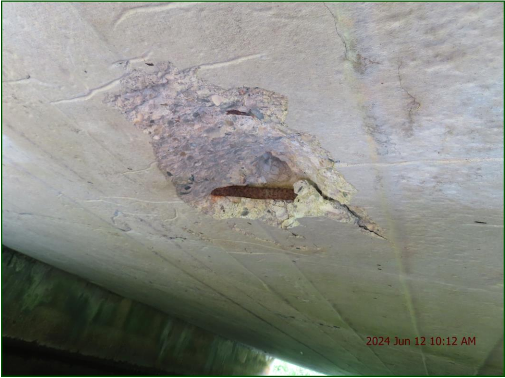
Description: Barrel: Severe localized spall with exposed reinforcing.
