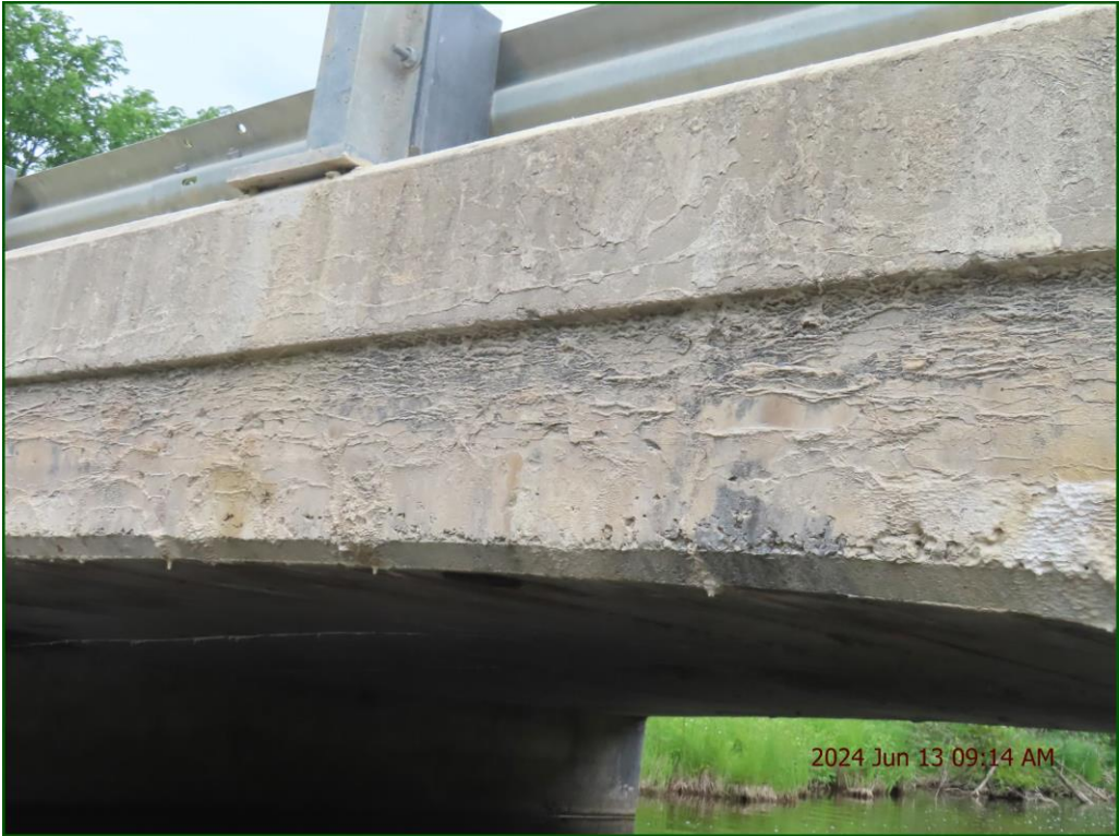
Description: Soffit (ext): Light to medium horizontal cracking with leachate staining.
