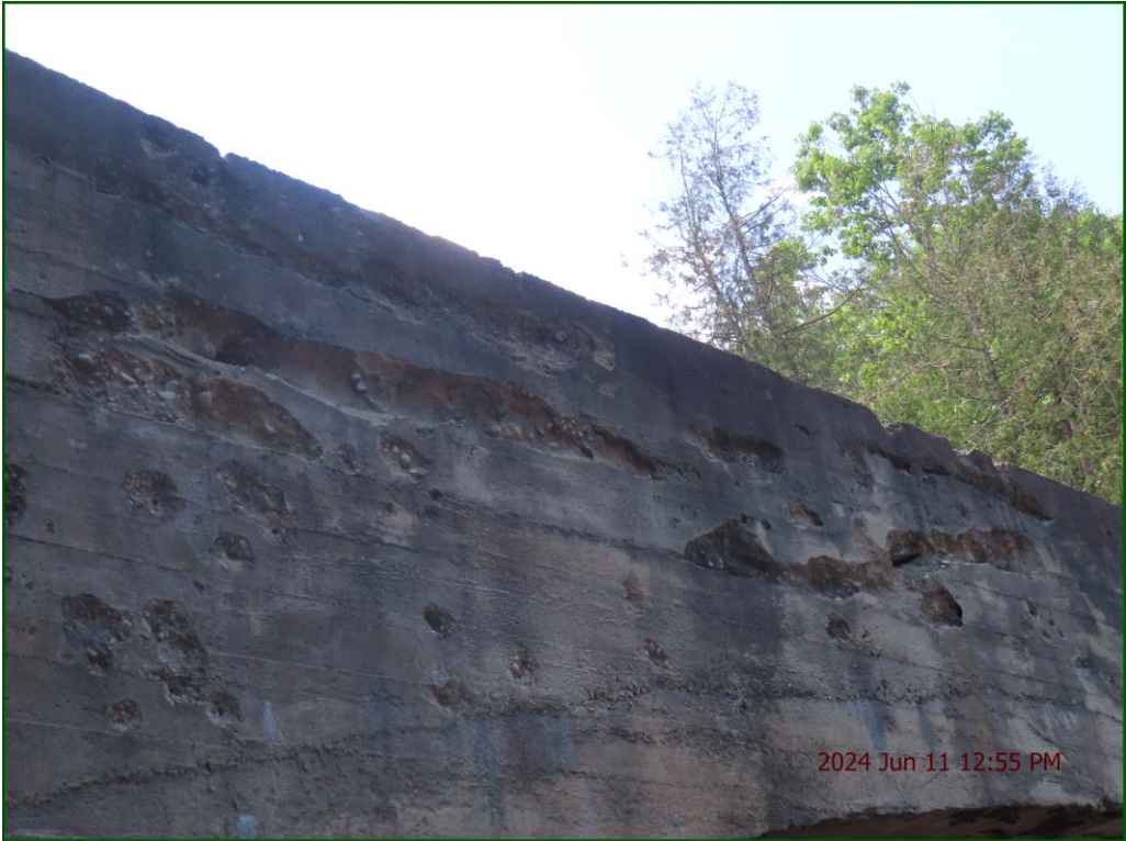
Description: Outlet: Severe spalling and disintegration throughout.
