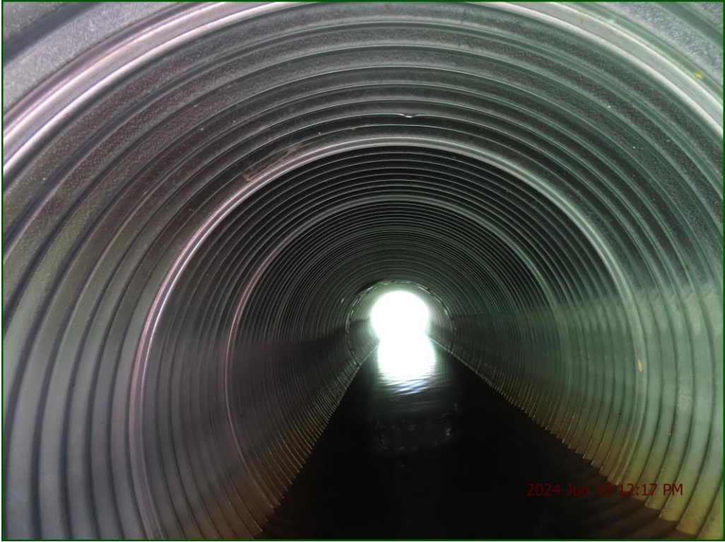
Description: Barrel: Minor deformations throughout.
