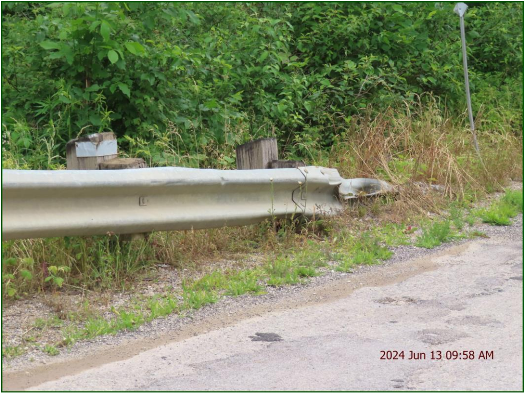
Description: Railing Systems: Severe rotting at SE quadrant.
