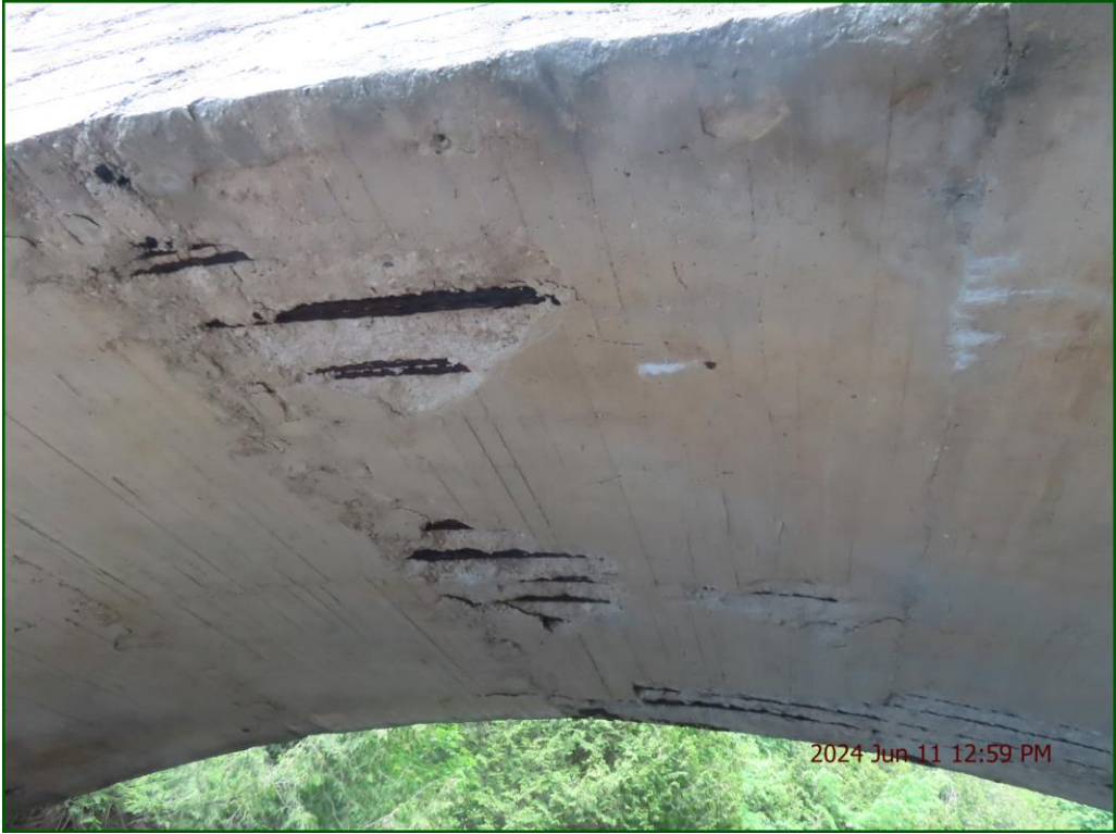
Description: Outlet: Severe spalling and disintegration throughout.
