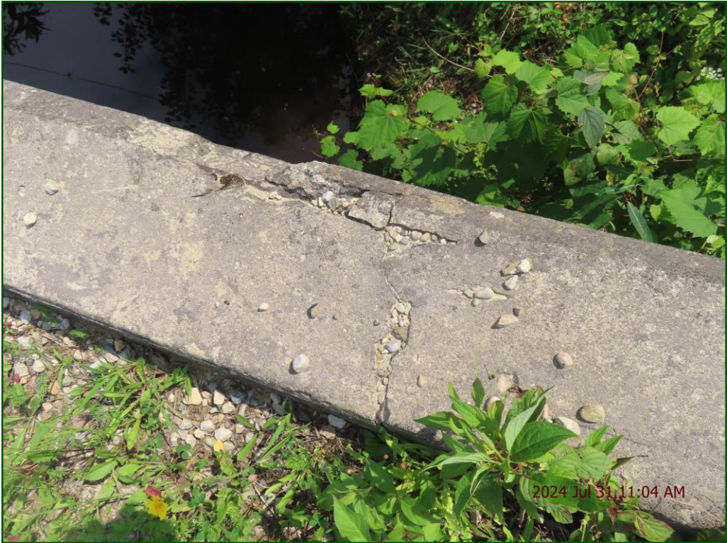
Description: Curbs: Wide cracking and spalling with exposed reinforcing.
