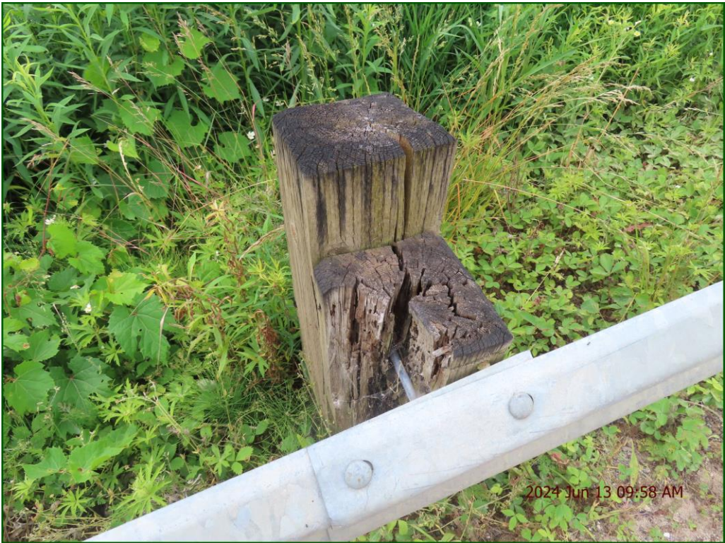
Description: Railing Systems: Severe rotting at SE quadrant.
