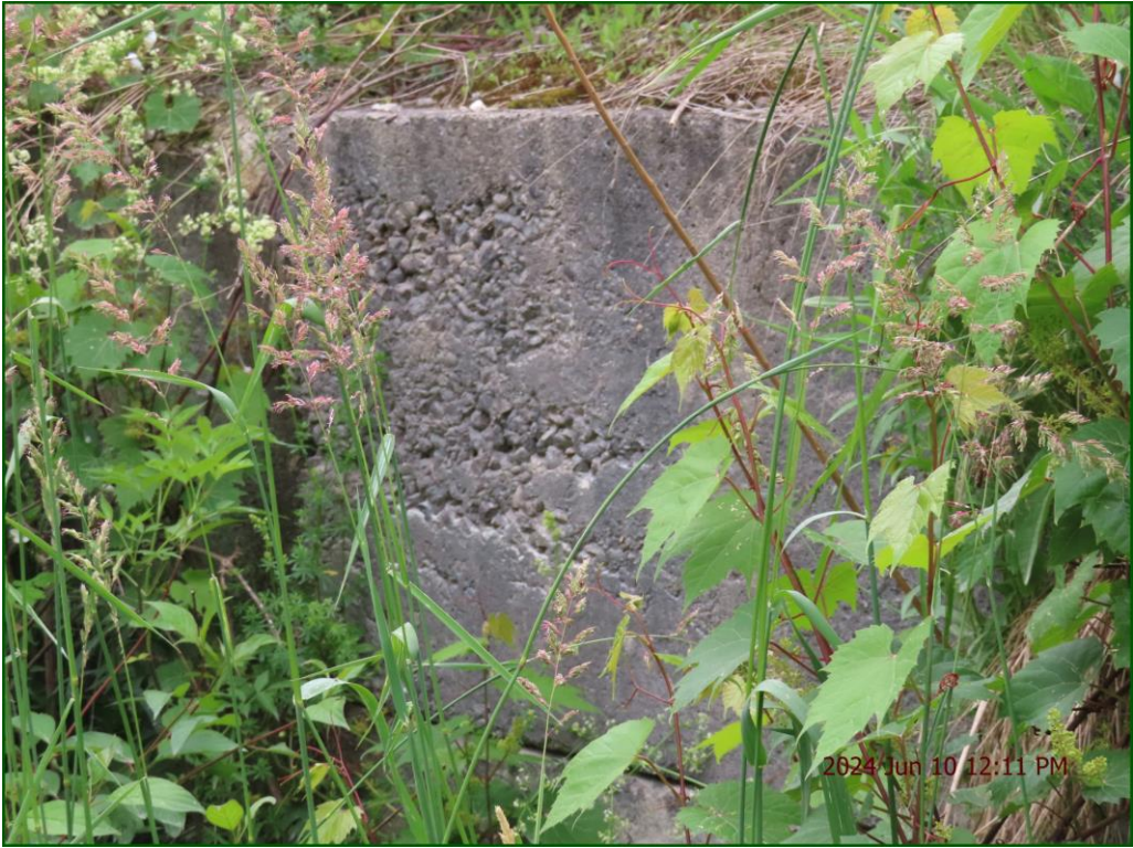
Description: Inlet: Light to medium honeycombing.
