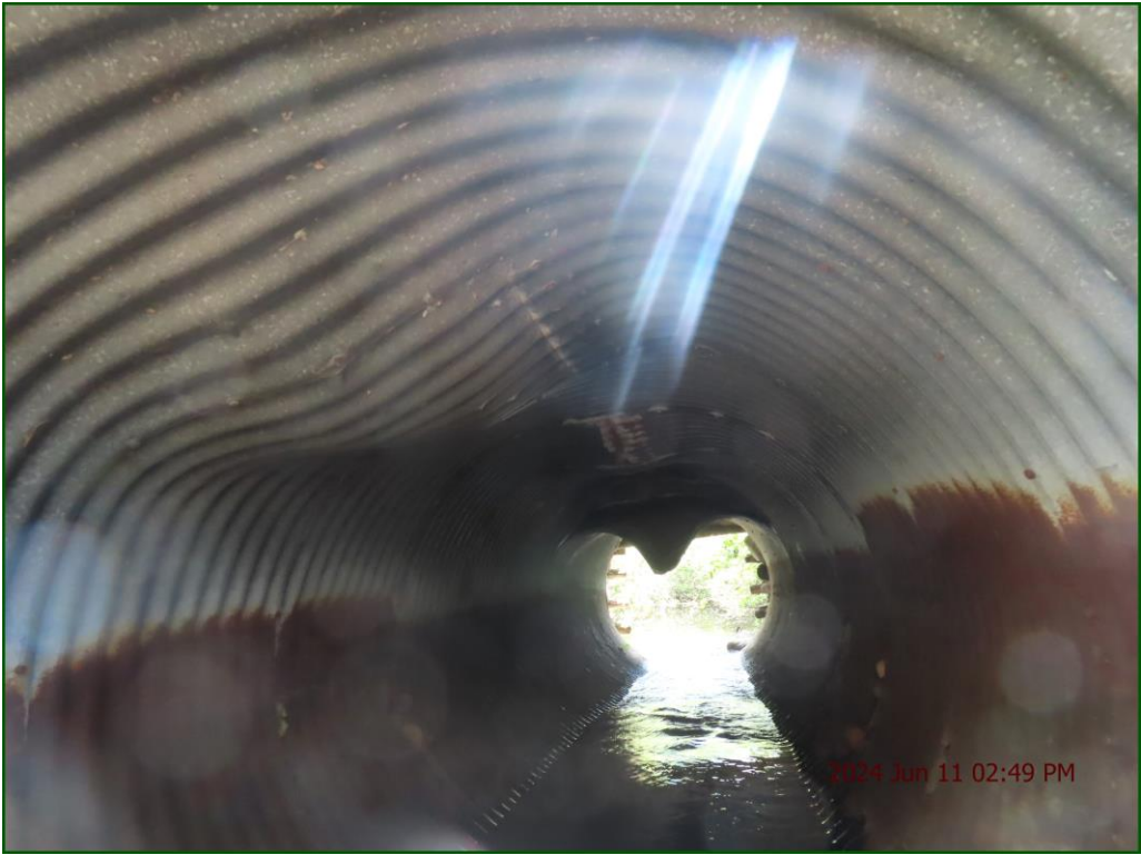
Description: Outlet: Minor scouring.
