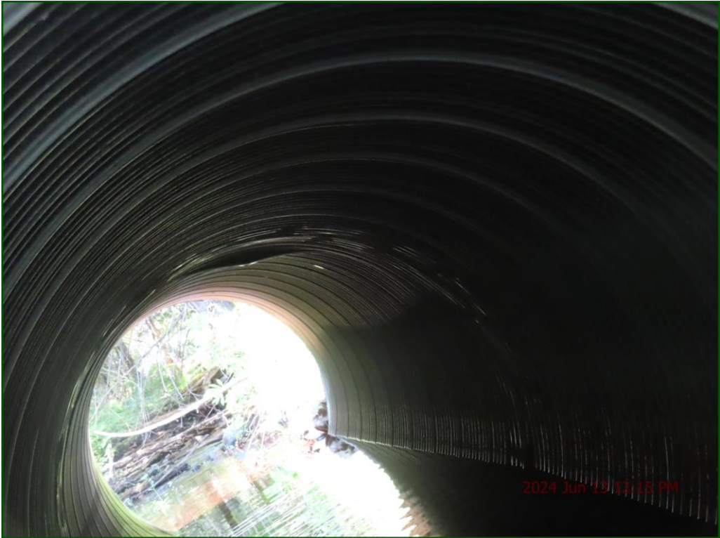
Description: Barrel: Minor deformations throughout.
