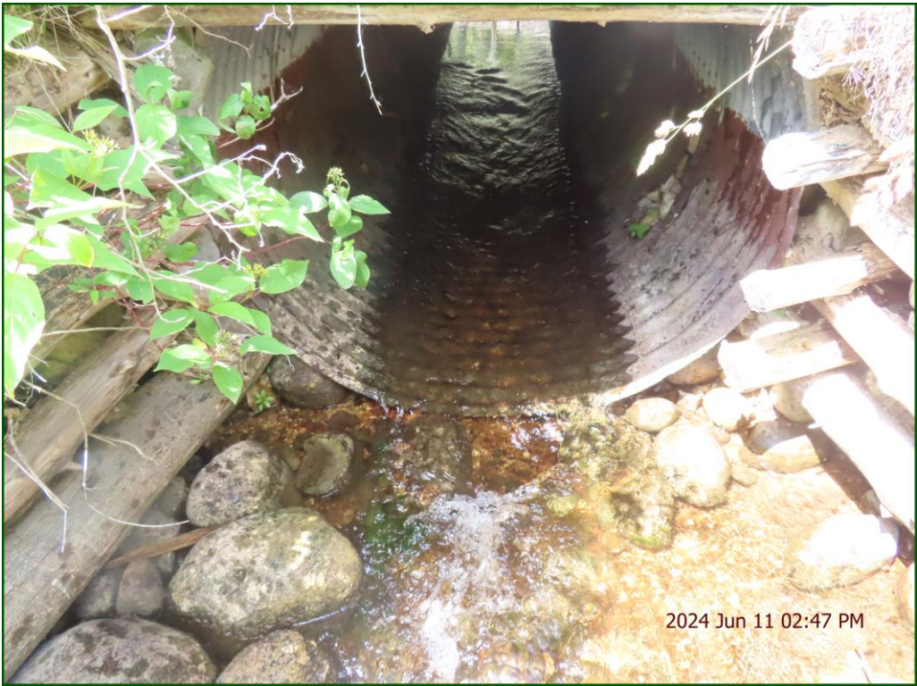
Description: Outlet: Minor scouring.
