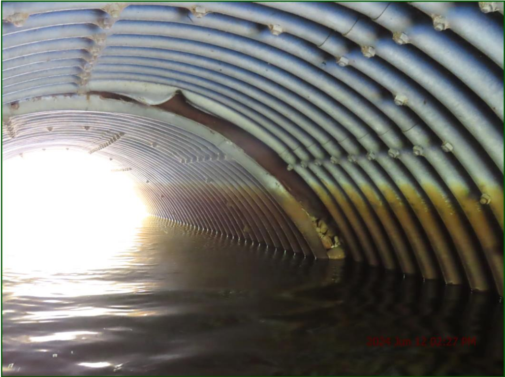
Description: Barrel: Separation of sections at mid point of south barrel.
