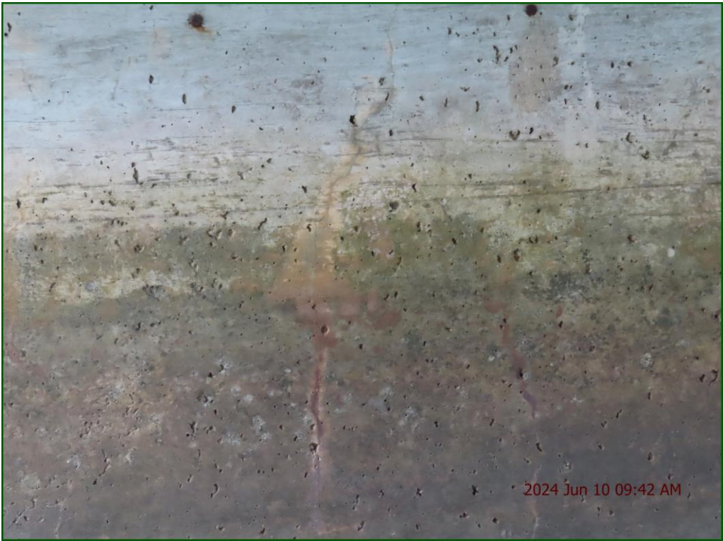
Description: Barrel: Light cracking and wetness staining.
