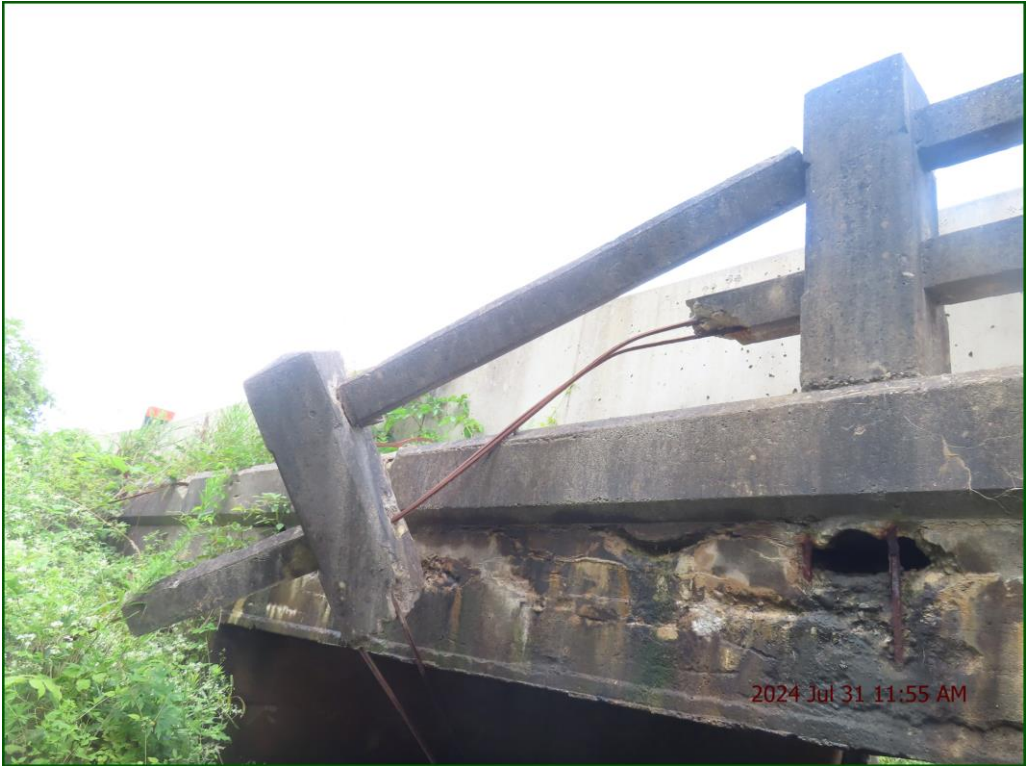
Description: Barrier/Parapet walls: Existing cast in place concrete barrier has failed.
