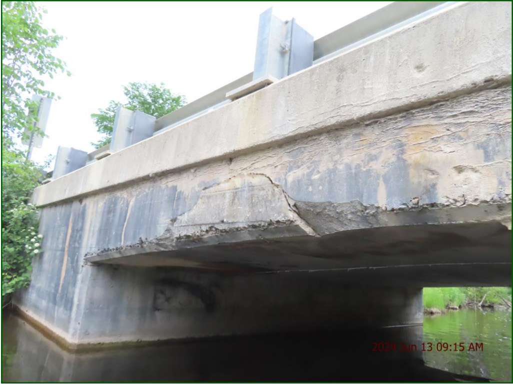
Description: Soffit (ext): Light to medium horizontal cracking with leachate staining.
