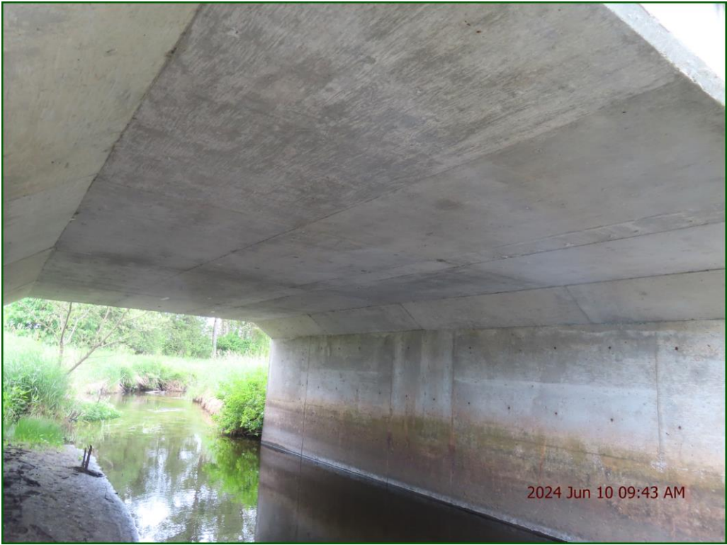
Description: Barrel: Light cracking and wetness staining.
