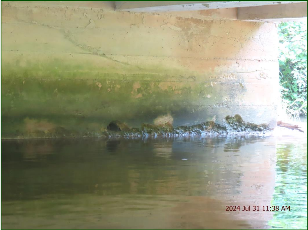
Description: Abutment Walls: Severe scouring and disintegration.
