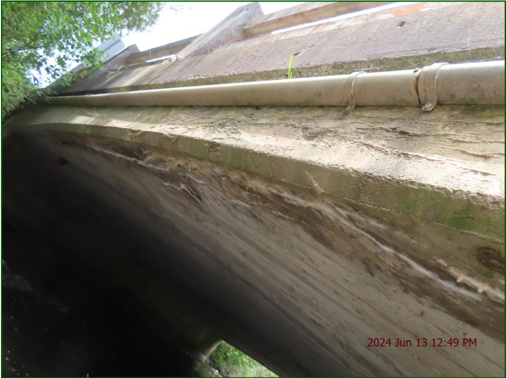
Description: Soffit (ext): Light to medium longitudinal cracking with leachate staining.
