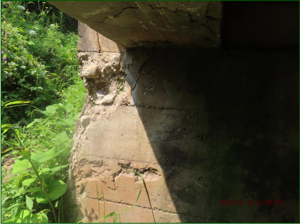
Description: Abutment Walls: Severe scouring and disintegration.
