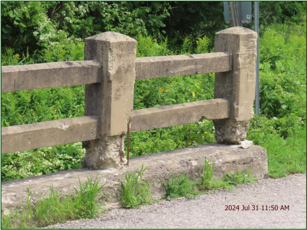
Description: Approach Railing System: Severe impact damage.
