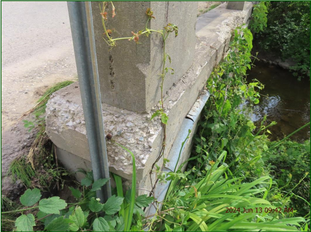
Description: Approach Curbs: Moderate disintegration on outside of SW approach.
