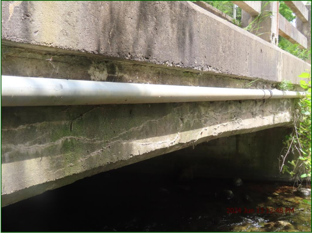
Description: Soffit (ext): Light to medium longitudinal cracking with leachate staining.
