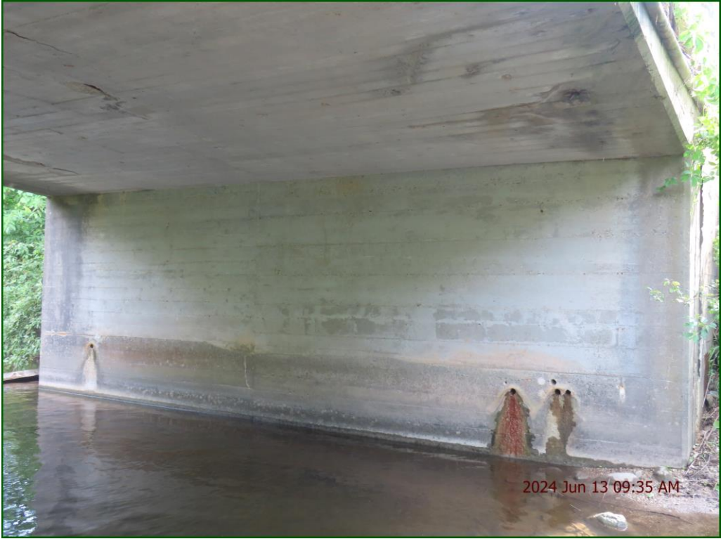
Description: Wingwalls: Light to medium vertical cracks throughout with leachate staining.
