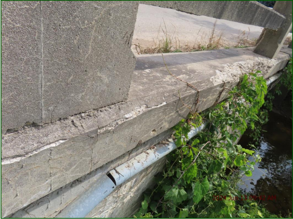
Description: Approach Curbs: Moderate disintegration on outside of SW approach.
