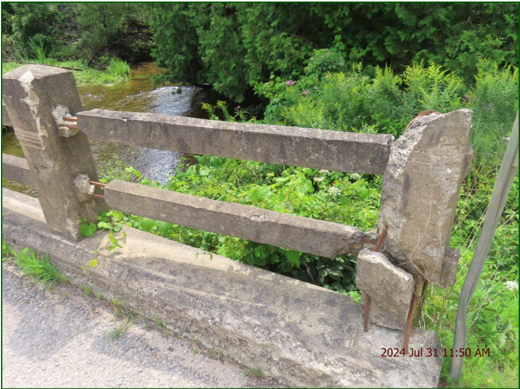
Description: Approach Railing System: Severe impact damage.
