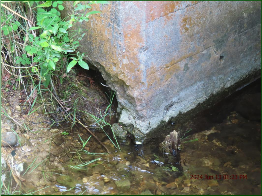
Description: Wingwalls: Severe spall on SW quadrant.
