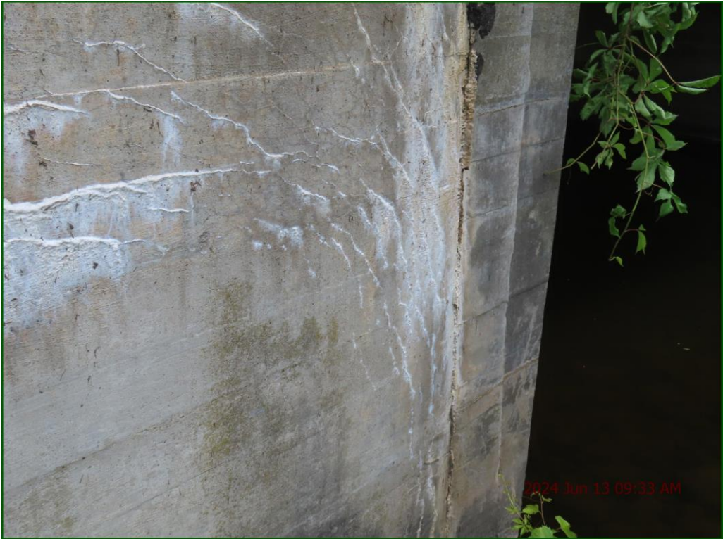
Description: Wingwalls: Light to medium vertical cracks throughout with leachate staining.
