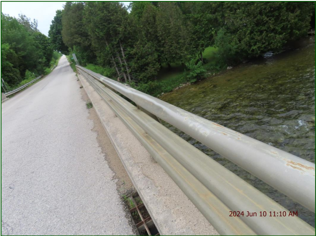
Description: Railing Systems: Minor impact damage.
