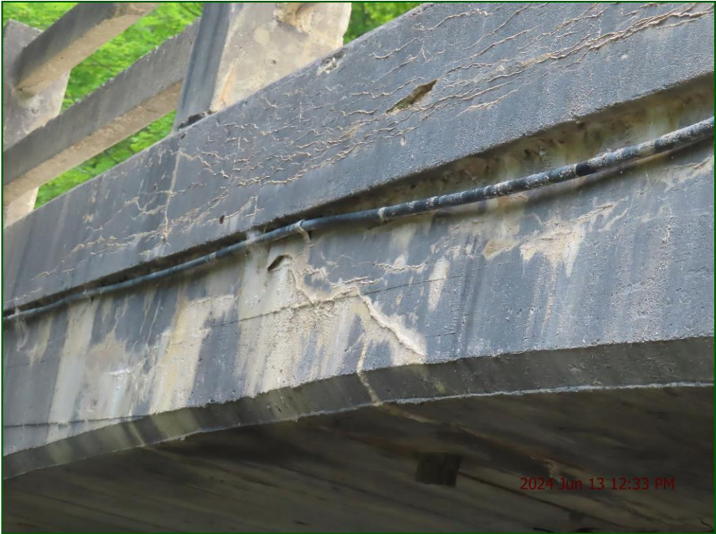
Description: Soffit (ext): Medium longitudinal cracking with leachate staining.
