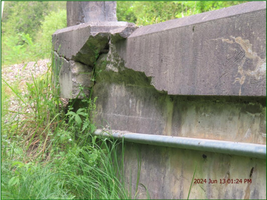
Description: Wingwalls: Severe spall on SW quadrant.
