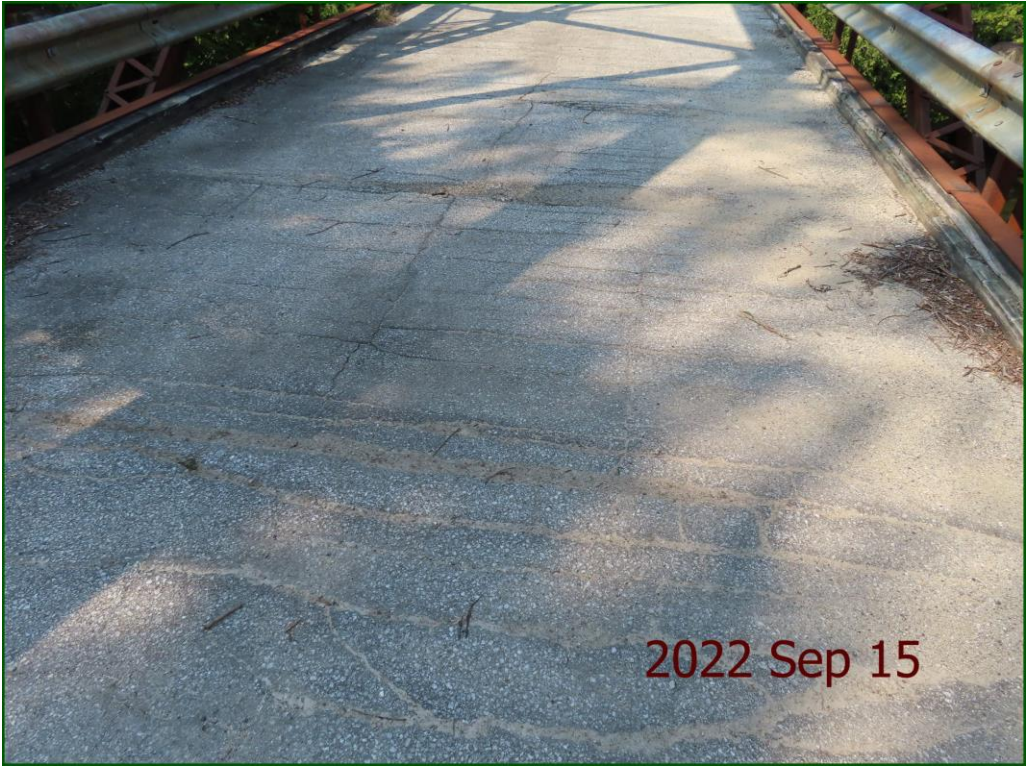
Description: Wearing surface: Medium to wide transverse cracks throughout.
