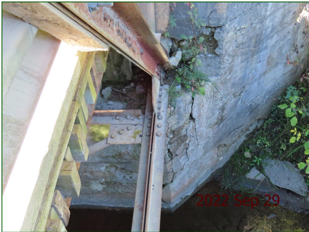
Description: Abutments: N-W Bearing seat cracking/crushing
