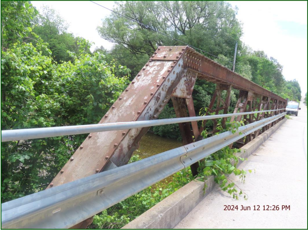
Description: Top chord: Areas of impact damage.
