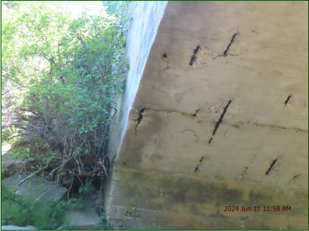
Description: Soffit (ext): Severe spalling with exposed reinforcing throughout (north) (3/3).
