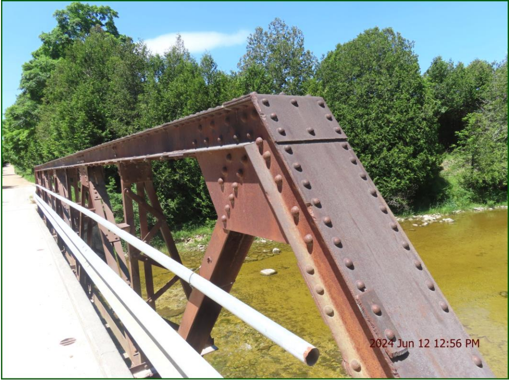
Description: Bottom chord: Medium to severe corrosion at NW with areas of 100% section loss.
