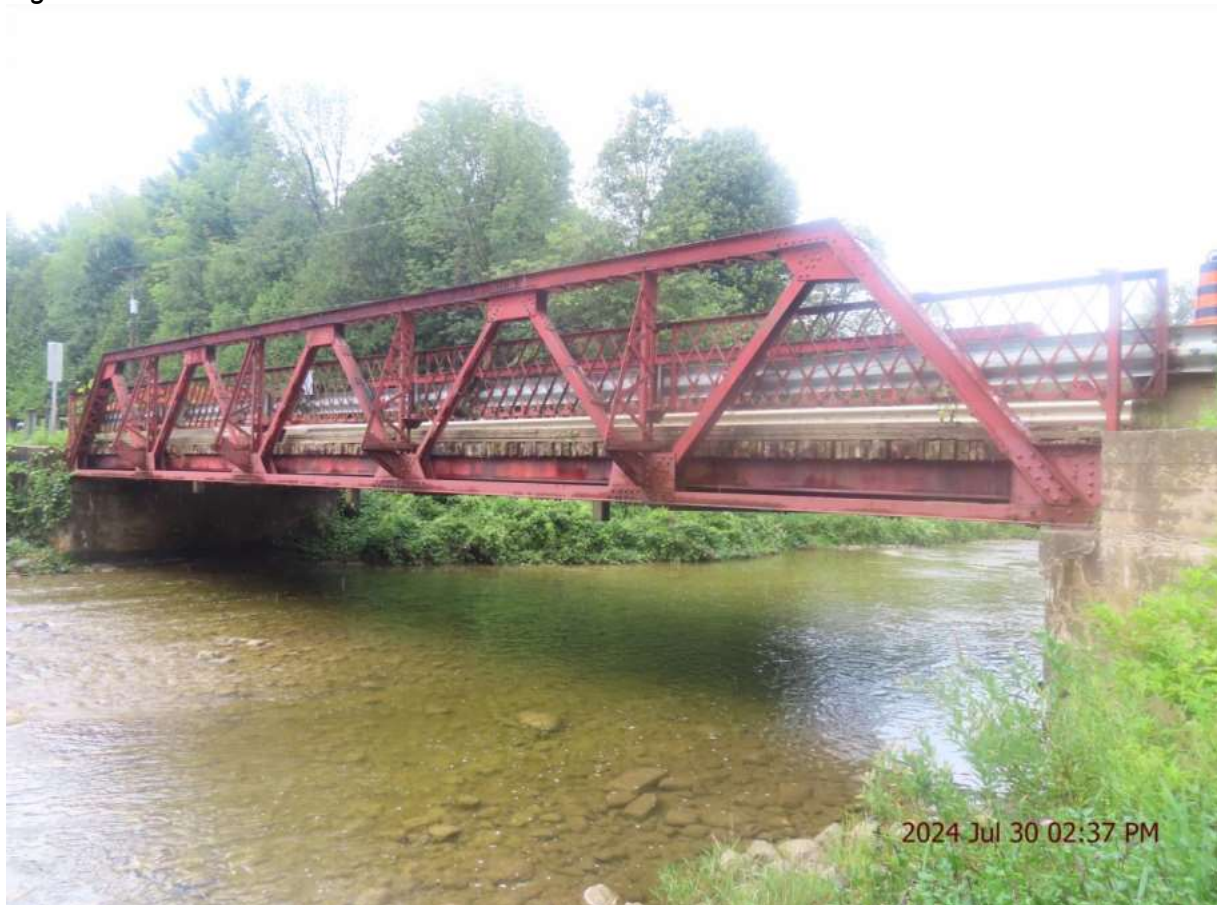
Figure 4.04: South Elevation View of Structure N-051
