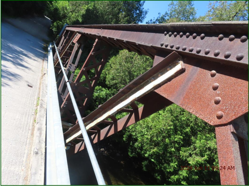
Description: Railing system: Severe rotting.
