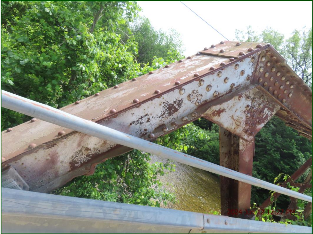
Description: Top chord: Areas of impact damage.
