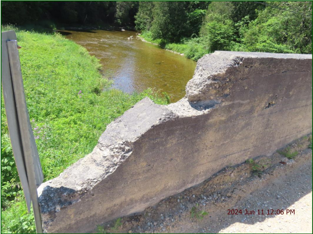
Description: Barrier/Parapet Walls: Severe spalling throughout.
