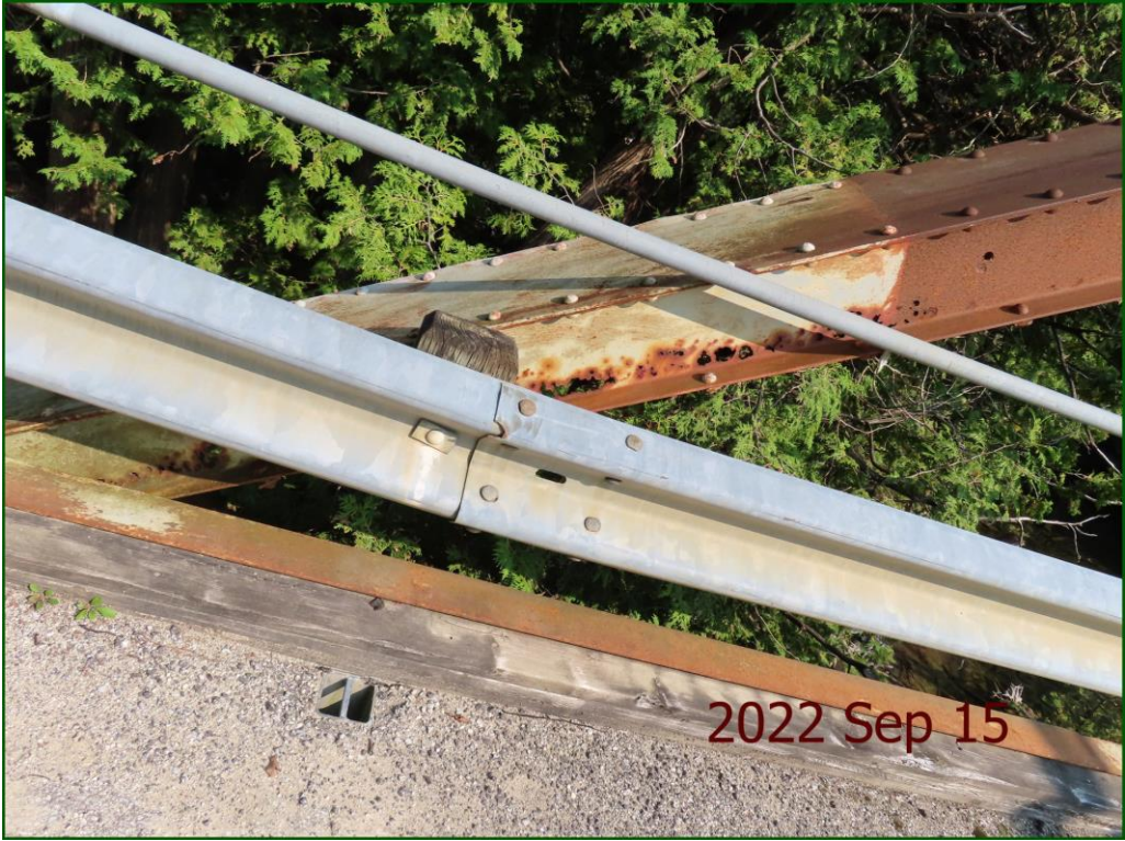
Description: Top chords: Areas of medium to severe corrosion with 100% section loss. (4/4)
