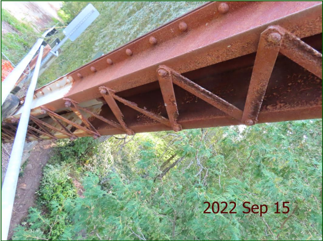
Description: Top chords: Areas of medium to severe corrosion with 100% section loss. (4/4)
