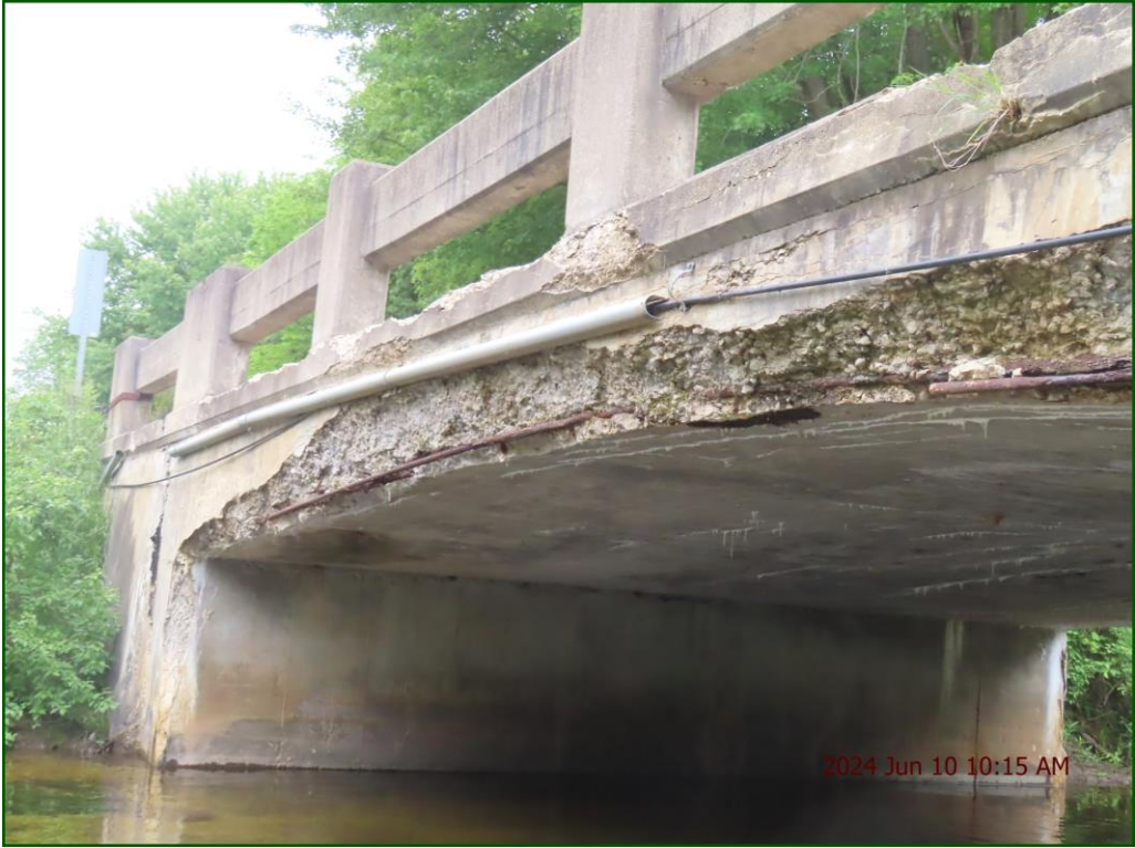
Description: Soffit (int): Medium to wide transverse and longitudinal cracking.
