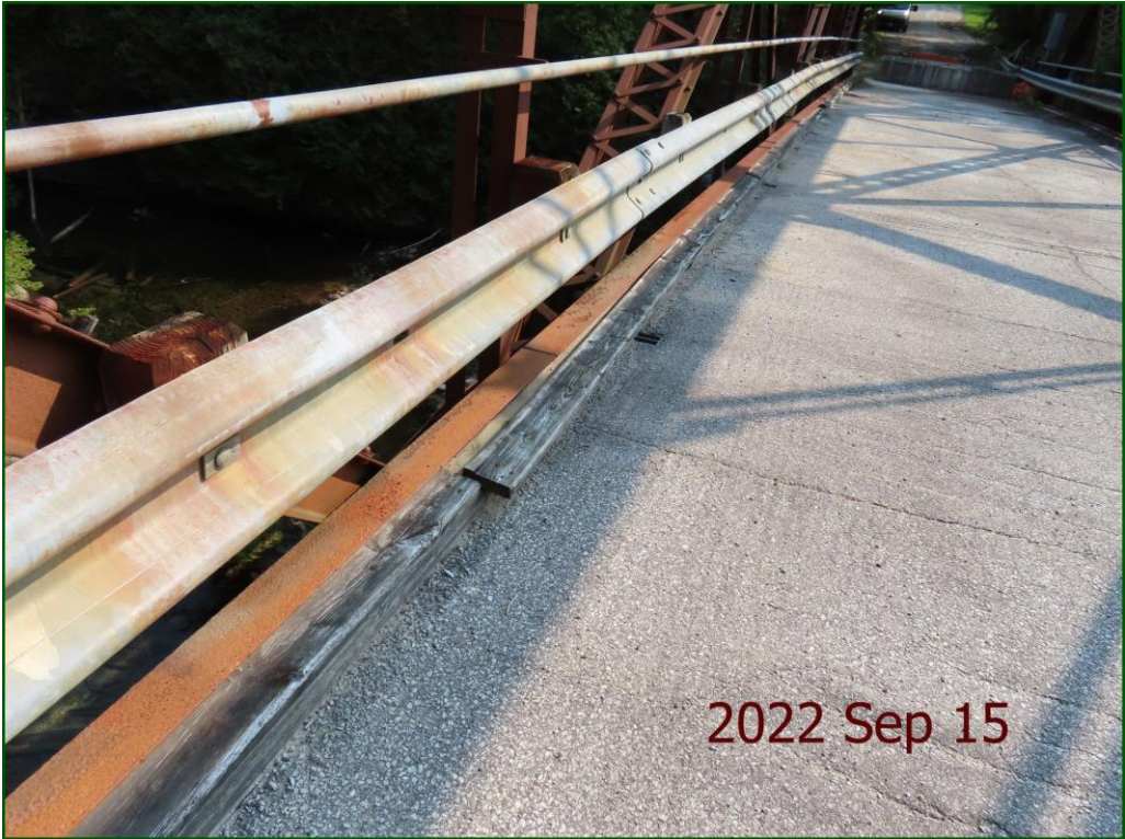
Description: Curbs: Impact damage throughout.
