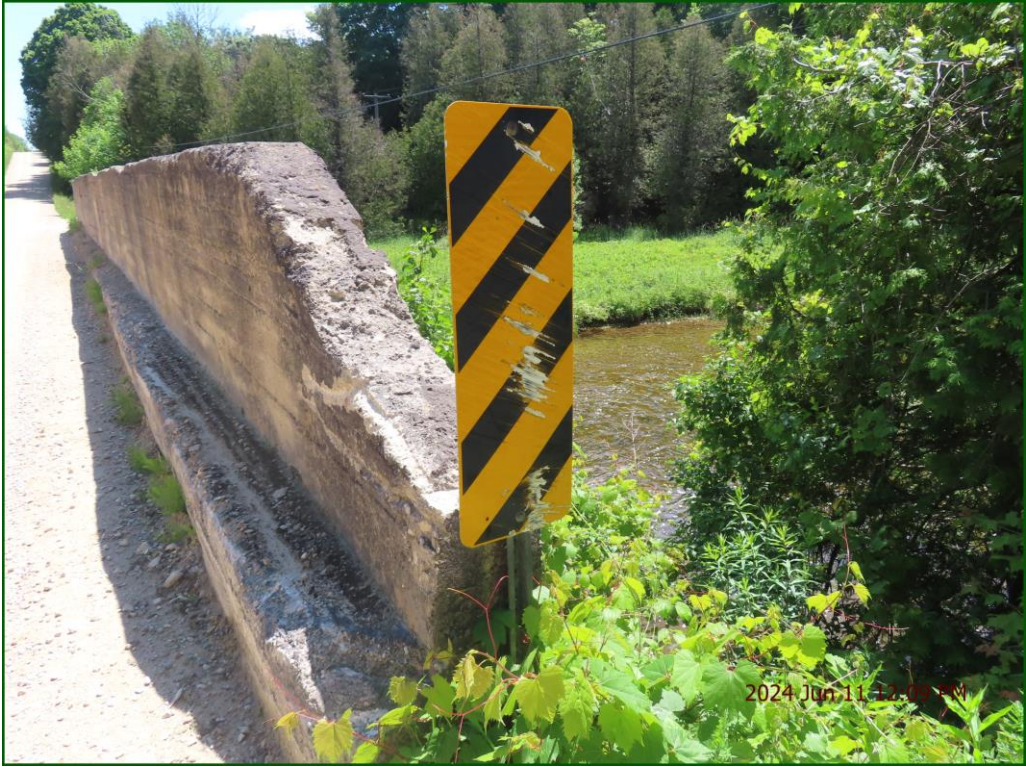
Description: Abutment Walls: Severe scouring.
