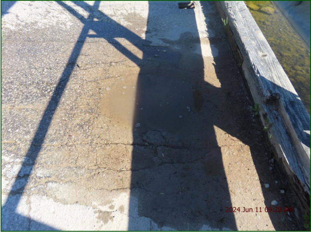
Description: Wearing surface: Severe pothole at midspan (2/4).
