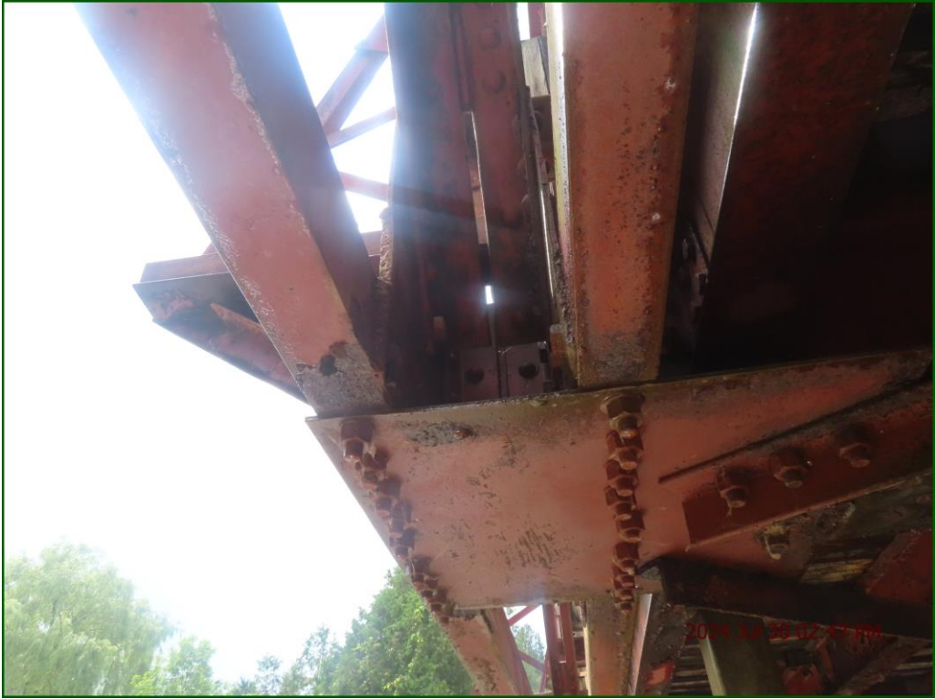
Description: Bottom Chord: Localized severe corrosion at bearing seats.
