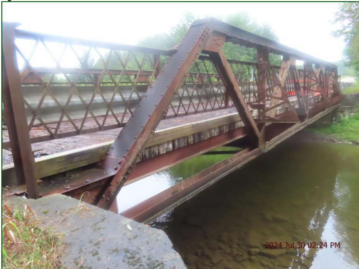
Figure 4.17: East Elevation View of Structure N-055
