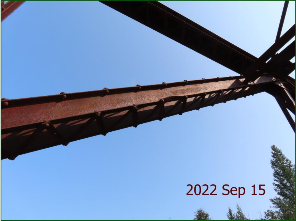
Description: Diagonals: Impact damage on various diagonals. (3/3)
