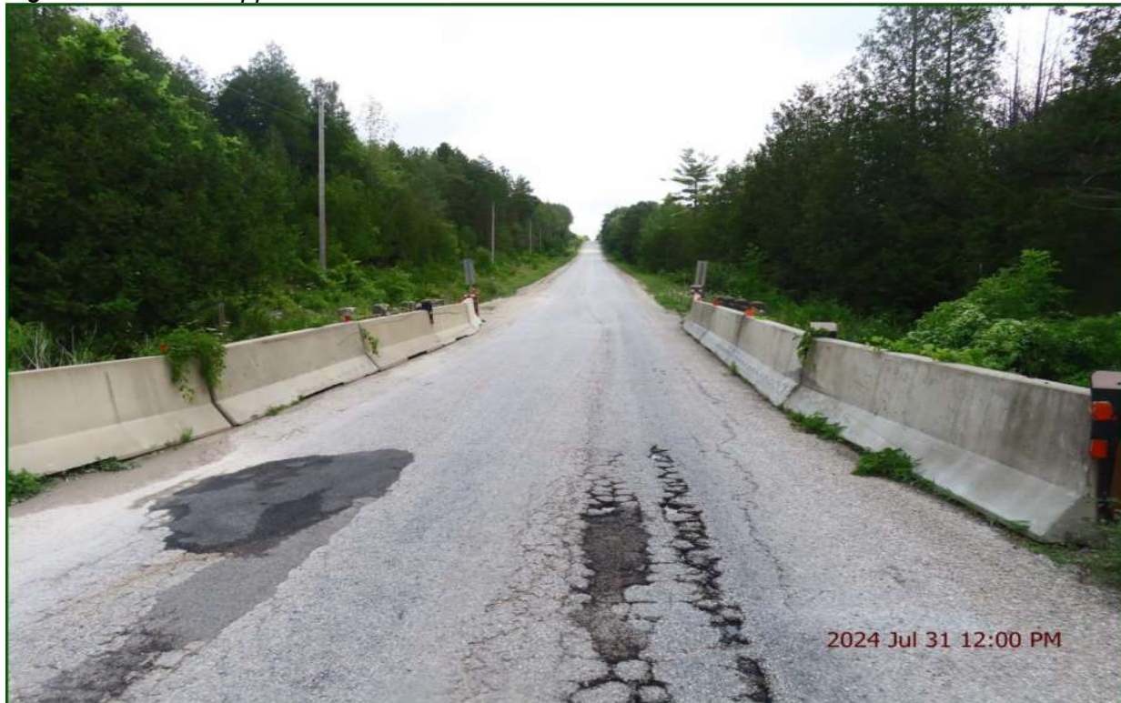
Figure 4.10: West Approach View of Structure N-060
