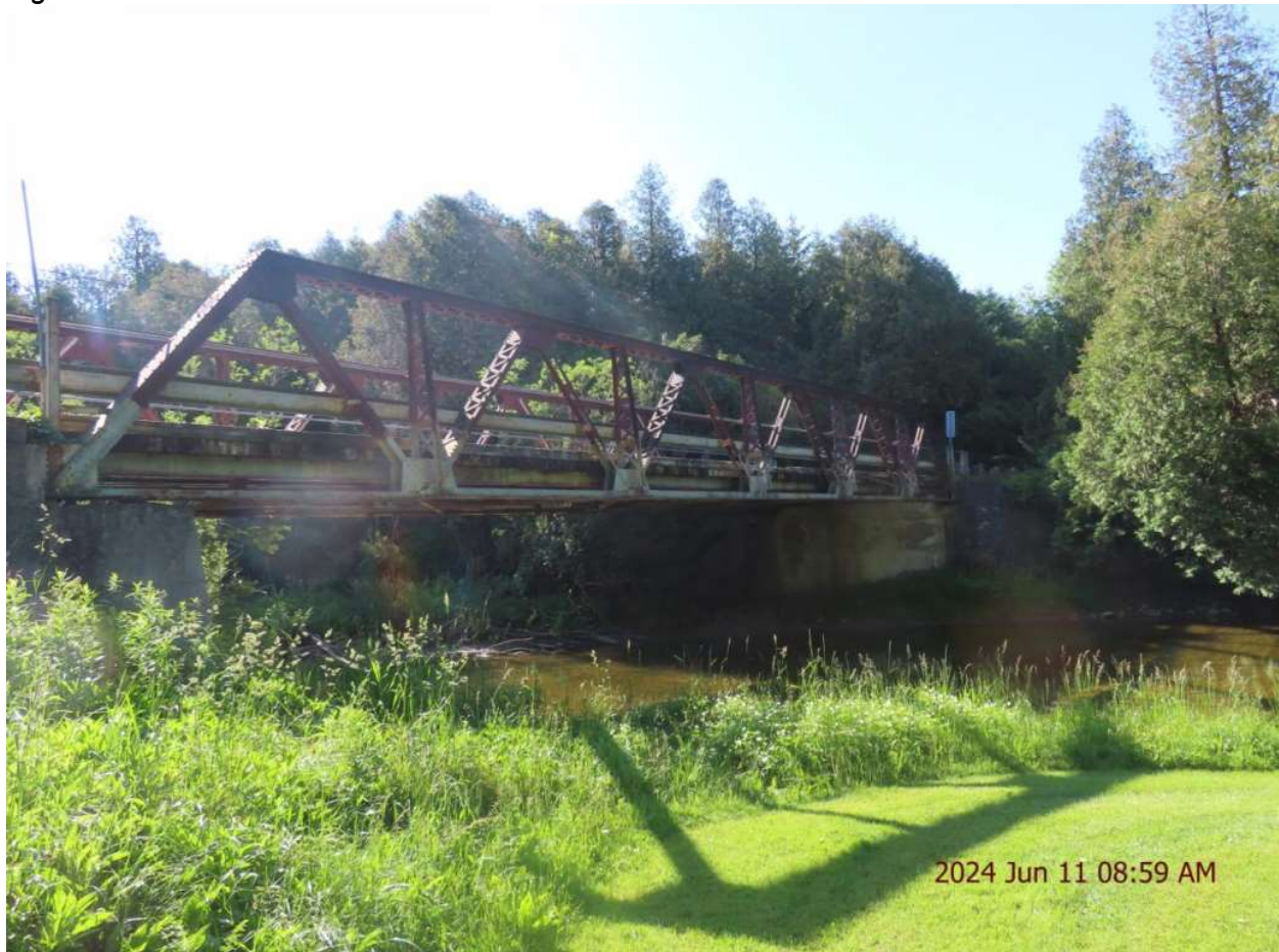
Figure 4.11: West Elevation View of Structure B-025
