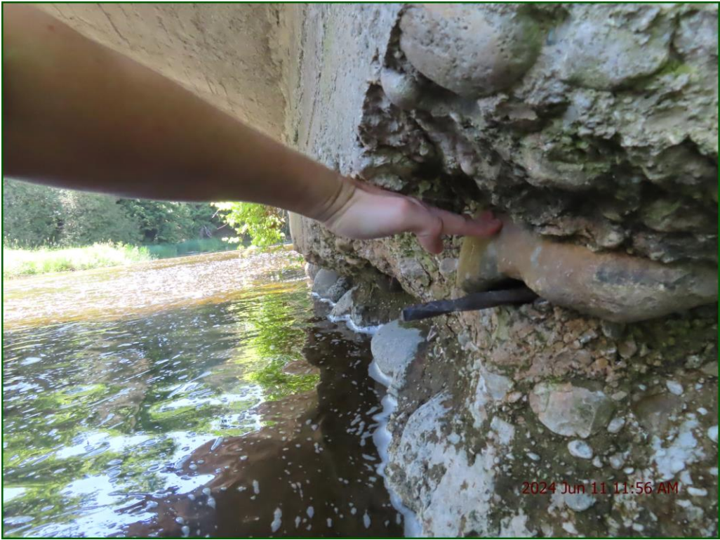
Description: Abutment Walls: Light to severe honeycombing throughout.
