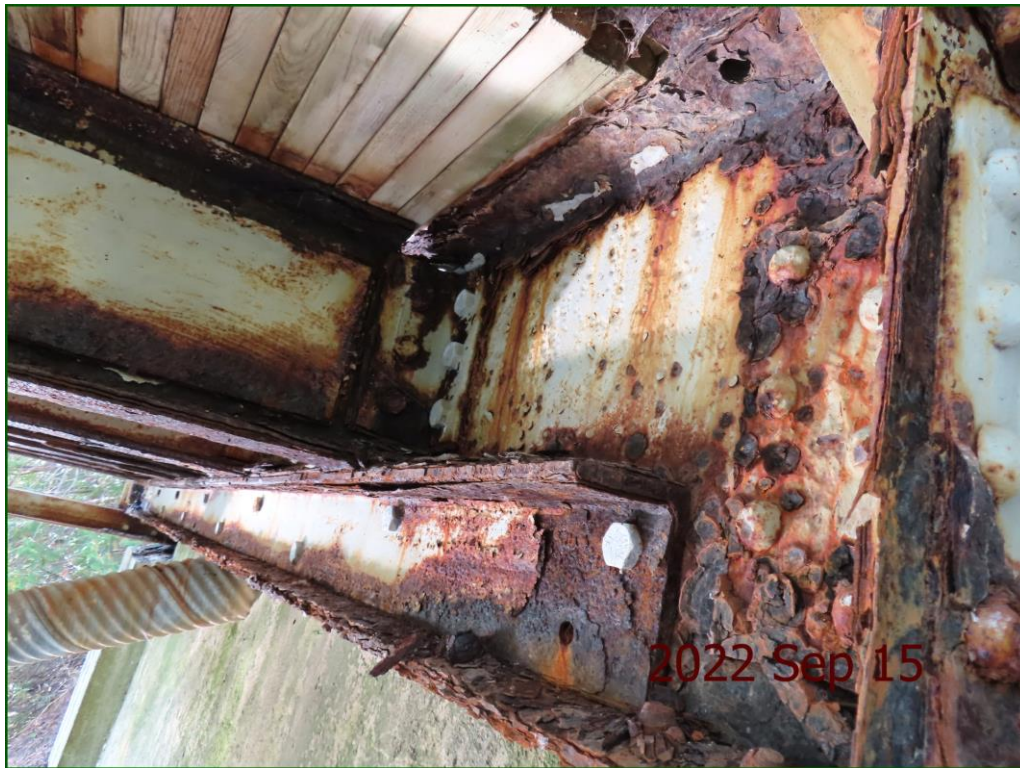
Description: Floor beams: Severe corrosion at ends. (2/3)
