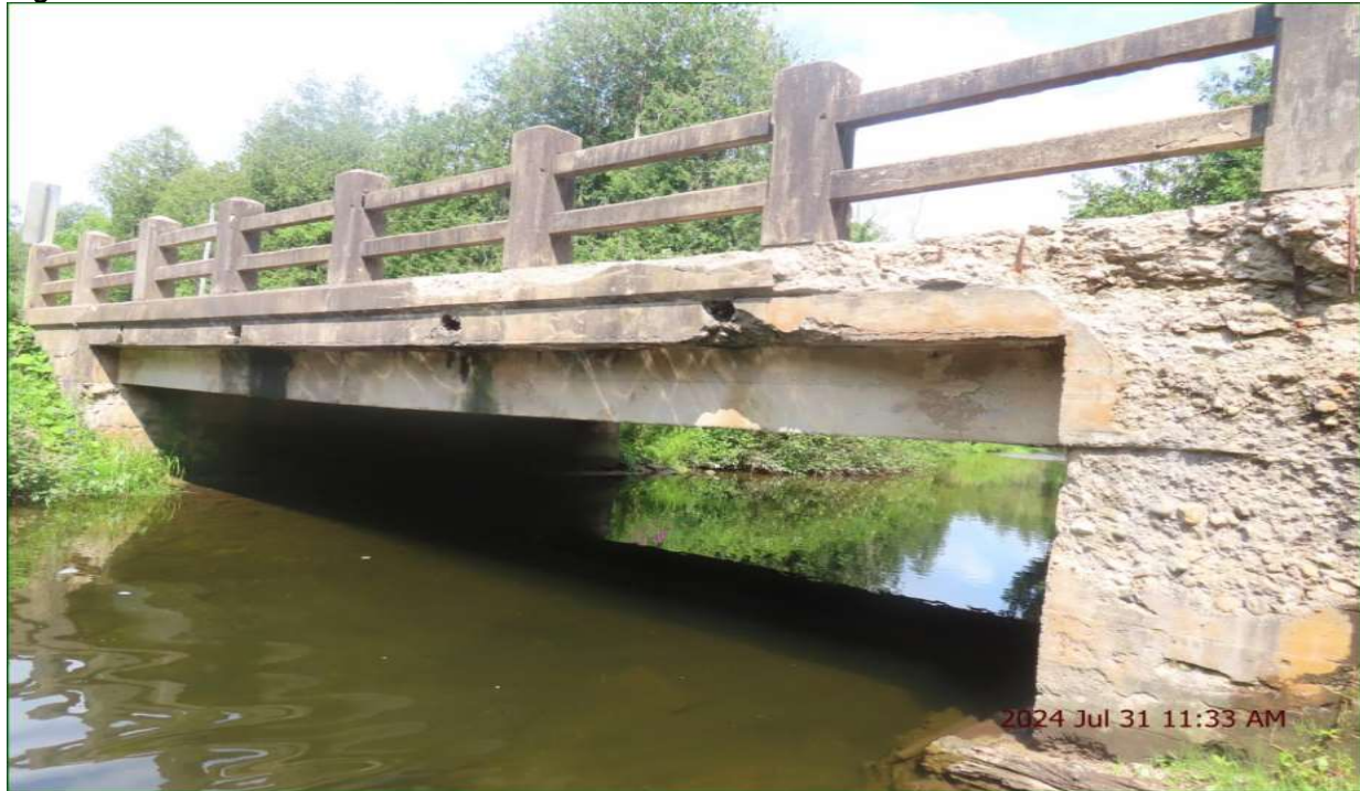
Figure 4.09: South Elevation View of Structure N-058
