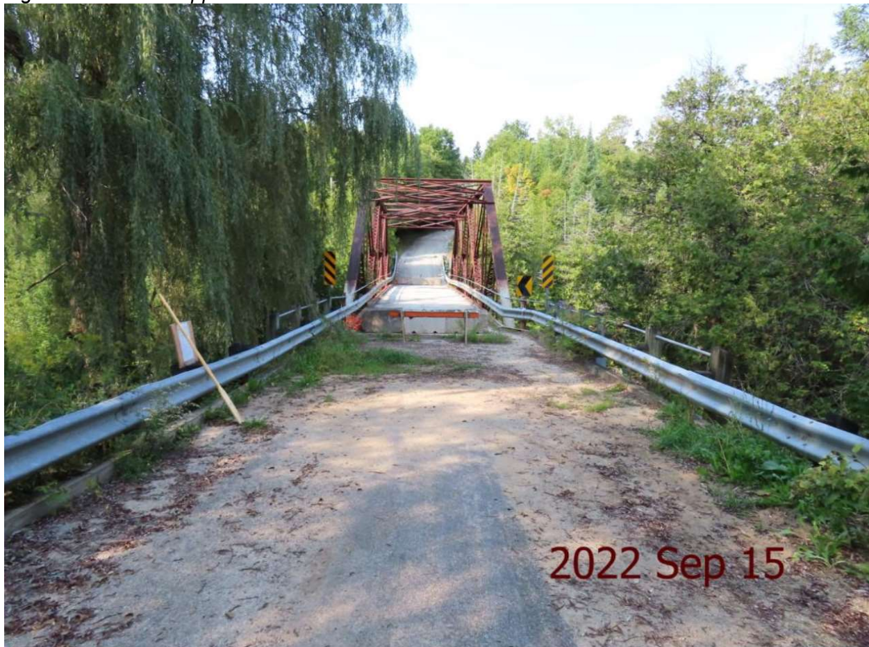
Figure 4.19: South Approach View of Structure G-033
