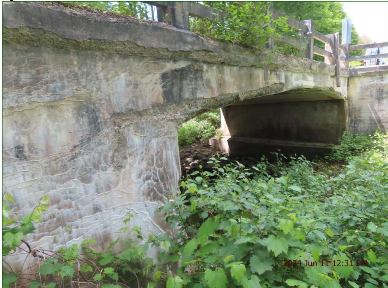
Figure 4.01: North Elevation View of Structure G-037
