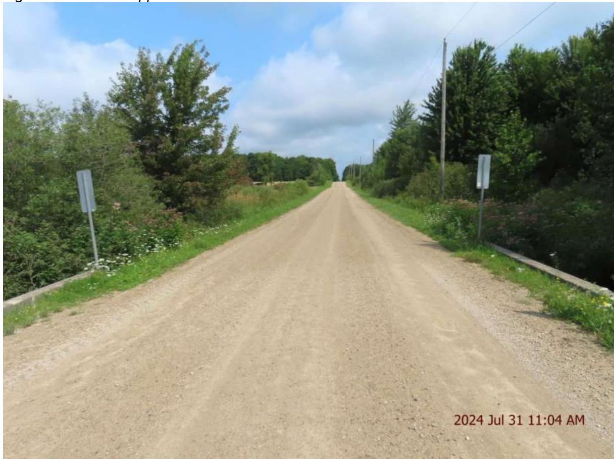
Figure 4.15: South Approach View of Structure N-185
