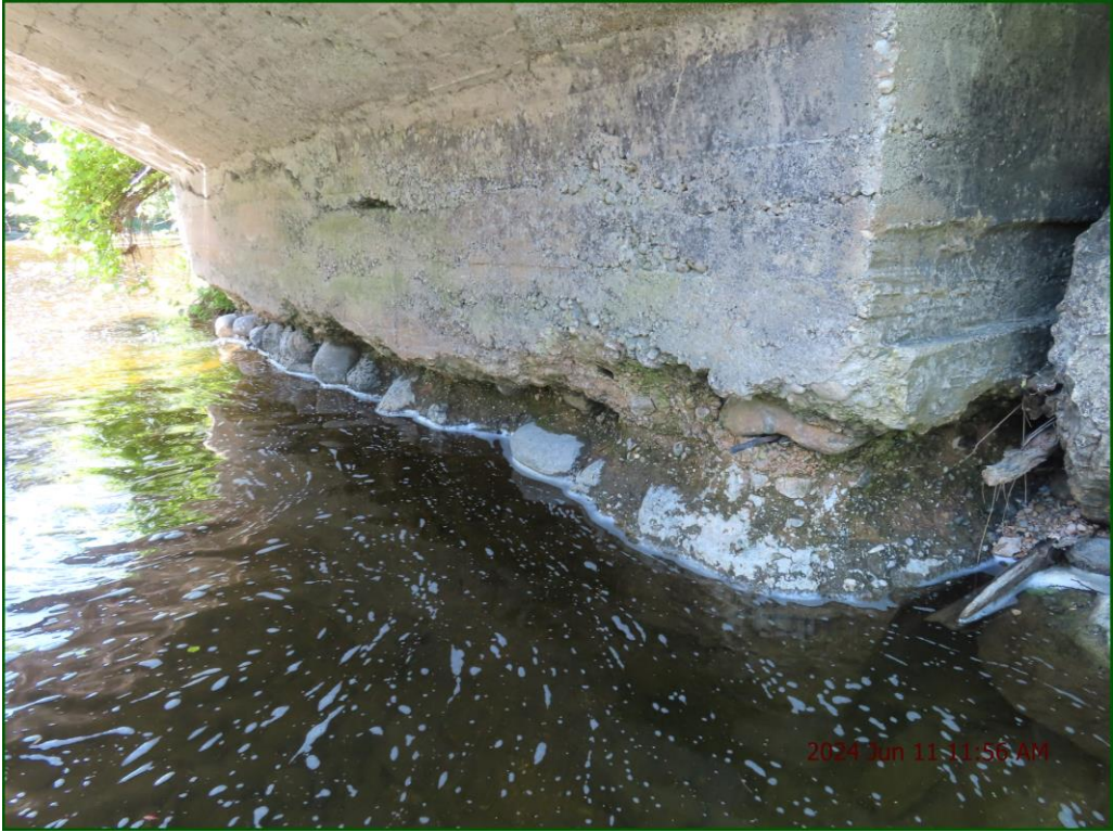
Description: Abutment Walls: Severe scouring and disintegration (2/3).
