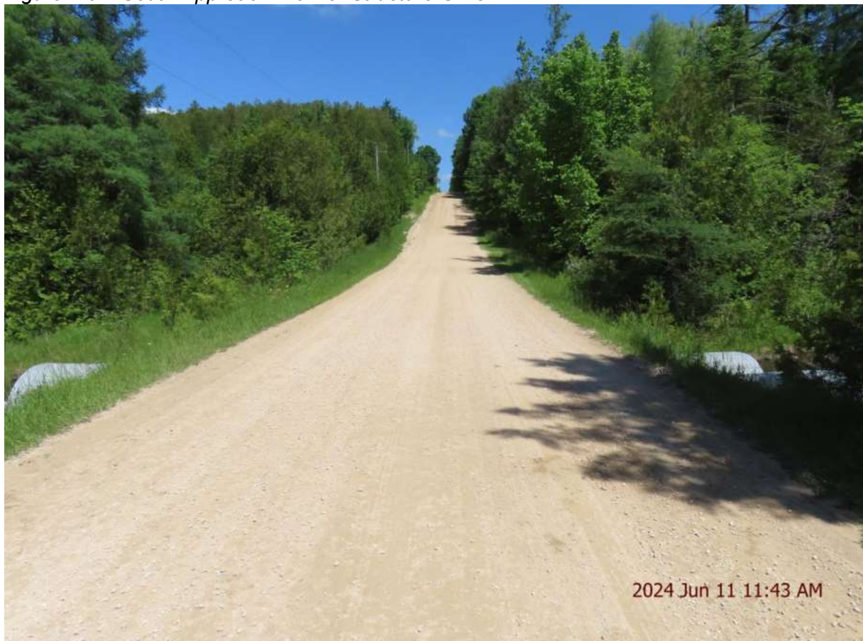
Figure 4.07: South Approach View of Structure G-132
