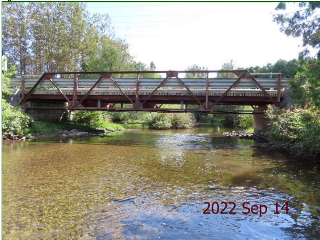
Figure 4.18: North Elevation View of Structure N-061
