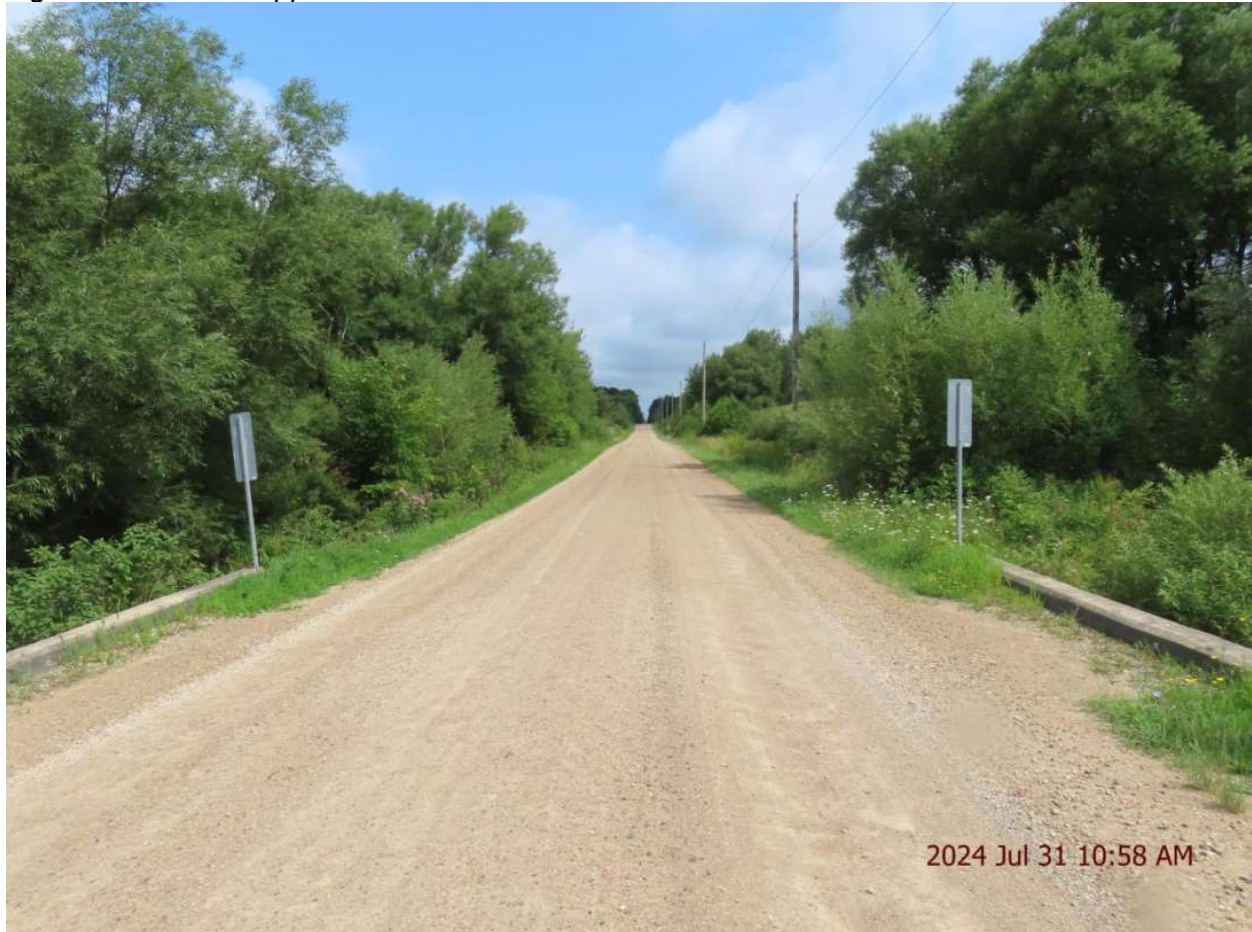
Figure 4.14: South Approach View of Structure N-184
