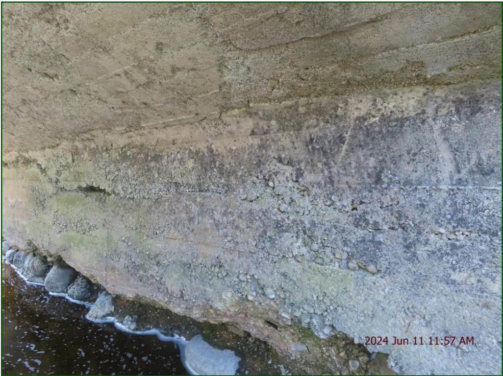
Description: Abutment Walls: Light to severe honeycombing throughout.
