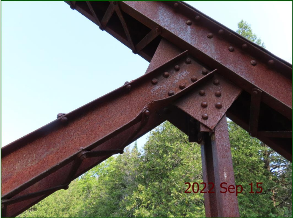
Description: Diagonals: Impact damage on various diagonals. (3/3)
