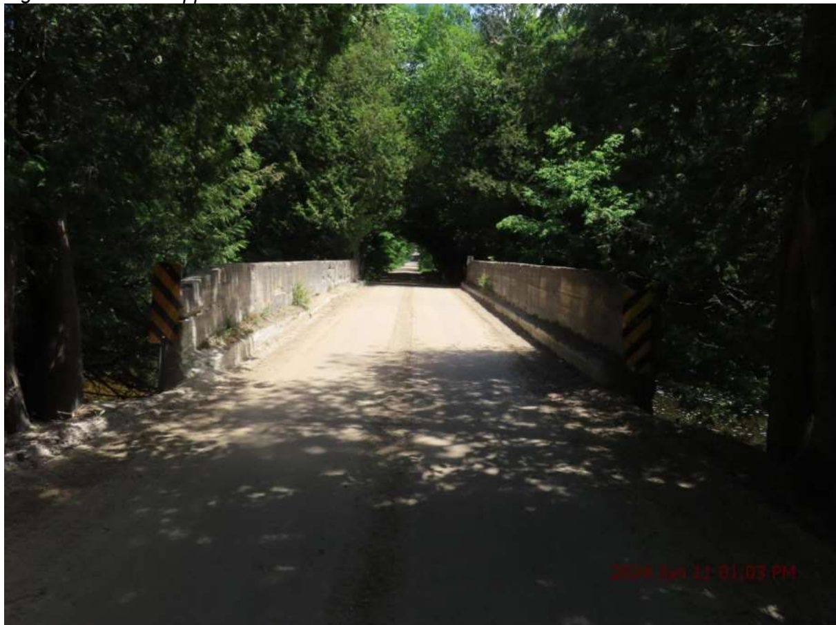
Figure 4.05: West Approach View of Structure G-044
