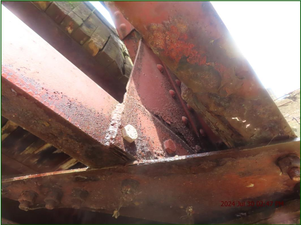
Description: Bottom Chord: Localized severe corrosion at bearing seats.
