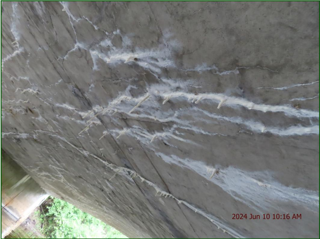
Description: Soffit (int): Medium to wide transverse and longitudinal cracking.
