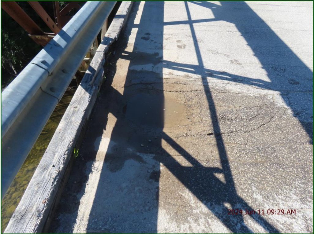
Description: Wearing surface: Severe pothole at midspan (2/4).
