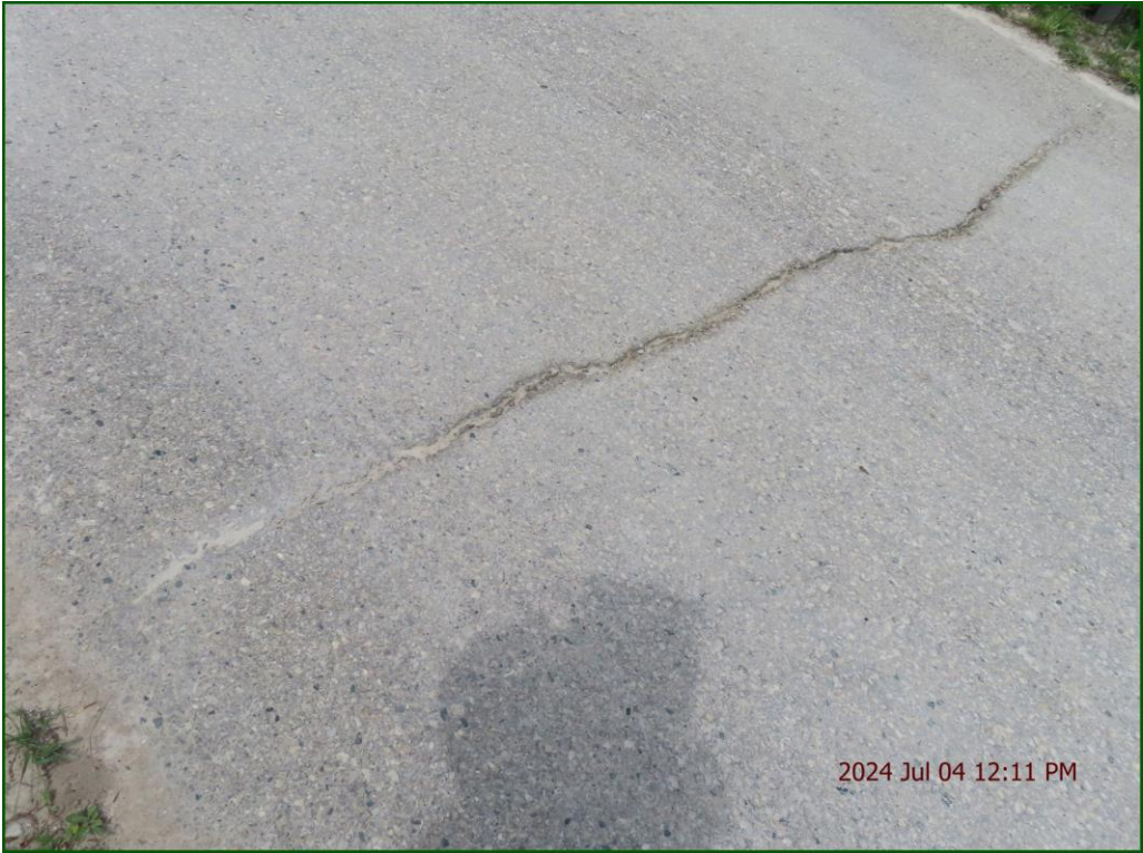
Description: Approach Wearing Surface: Wide transverse crack.
