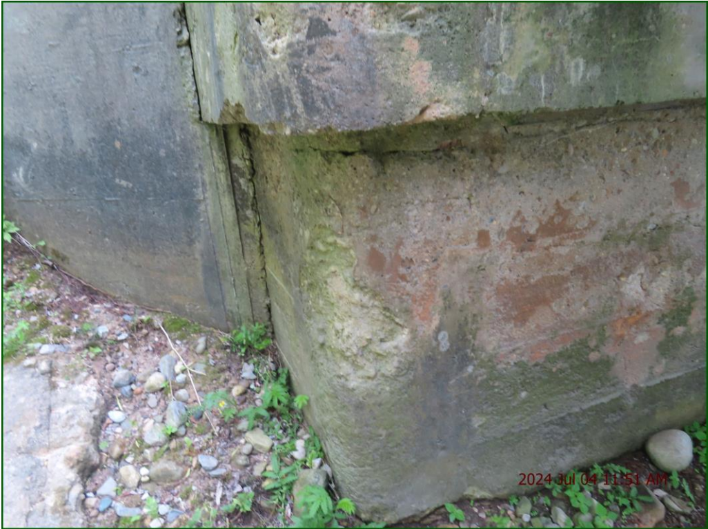
Description: Abutment Walls: Light to severe spalling throughout.
