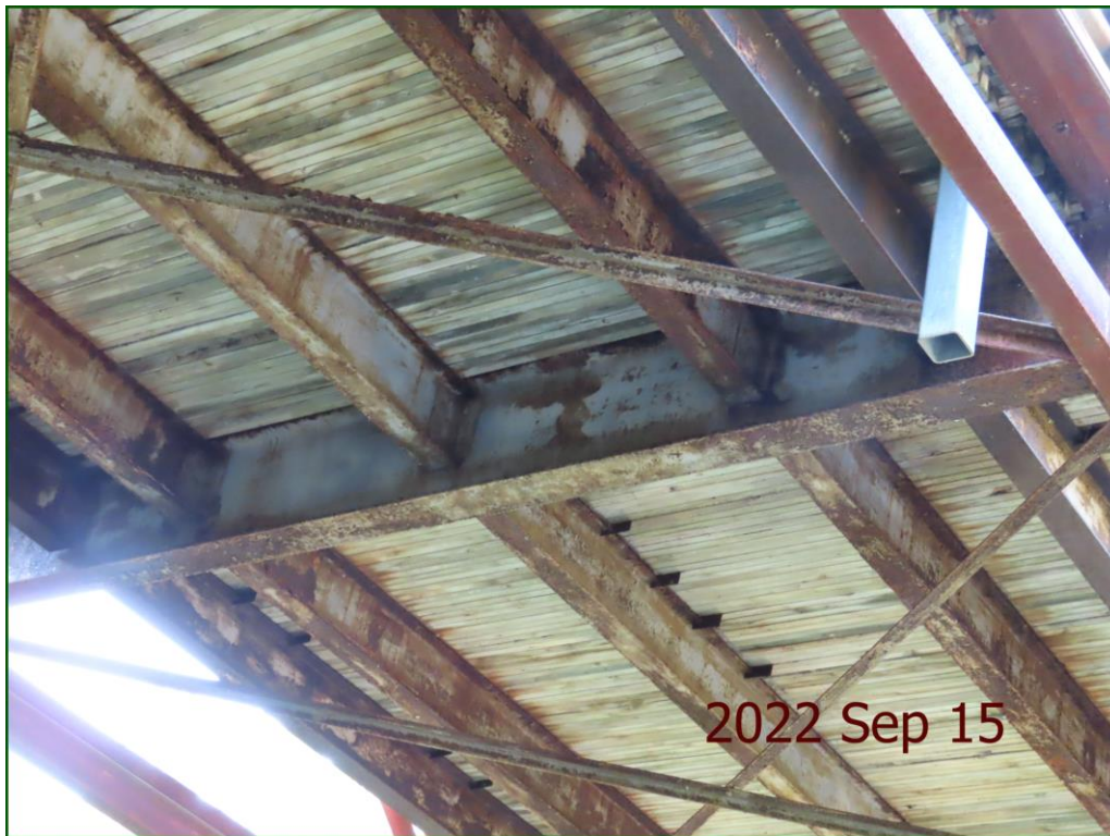
Description: Floor beams: Severe corrosion at ends. (2/3)
