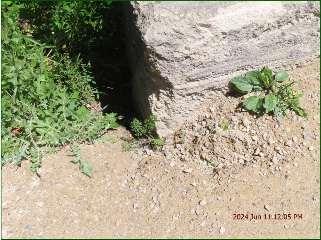
Description: Barrier/Parapet Walls: Severe spalling throughout.
