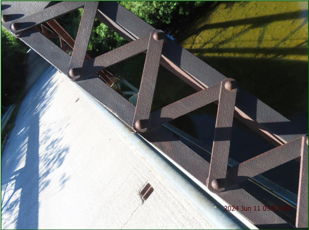
Description: Verticals/diagonals: Railing system welded to structure.
