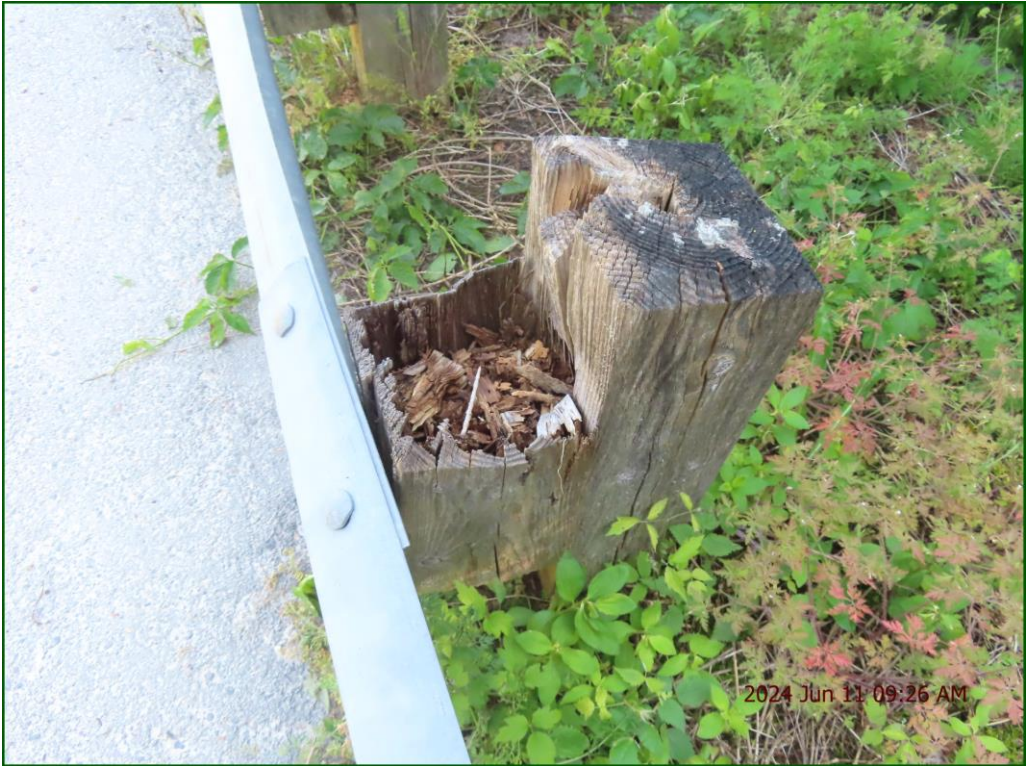
Description: Railing system: Severe rotting.
