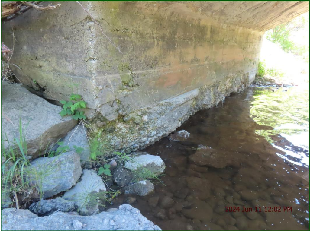
Description: Abutment Walls: Severe scouring.
