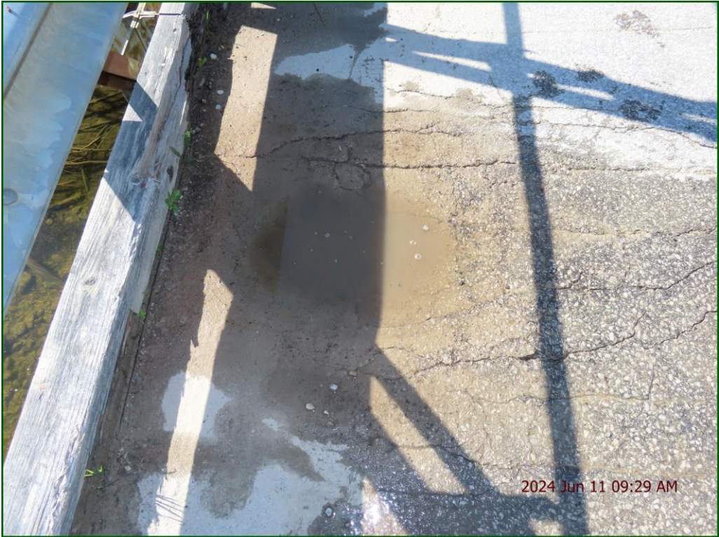
Description: Wearing surface: Severe pothole at midspan (4/4).
