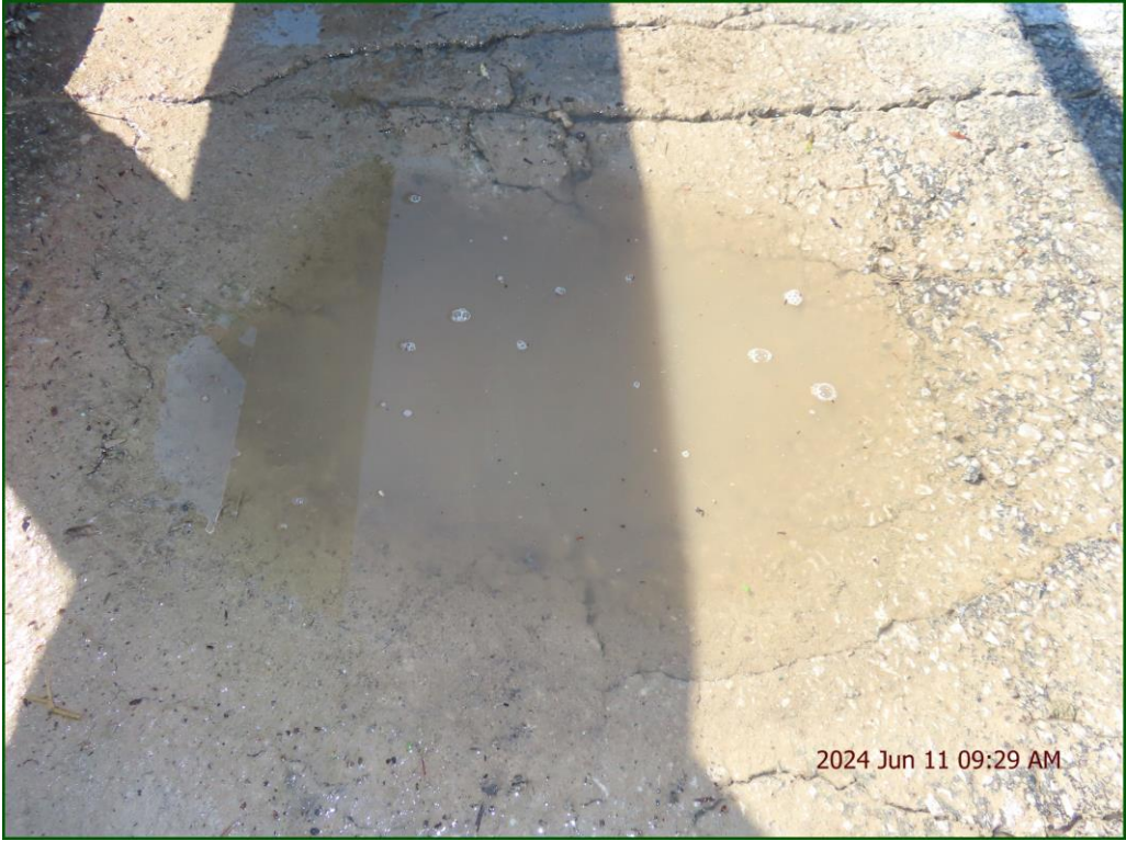
Description: Wearing surface: Severe pothole at midspan (4/4).
