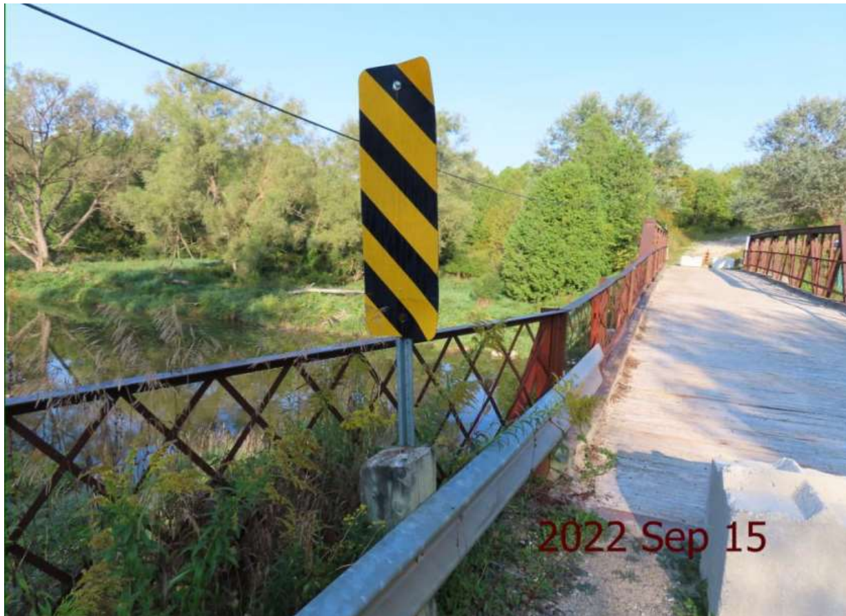
Figure 4.20: South Approach View of Structure N-070
