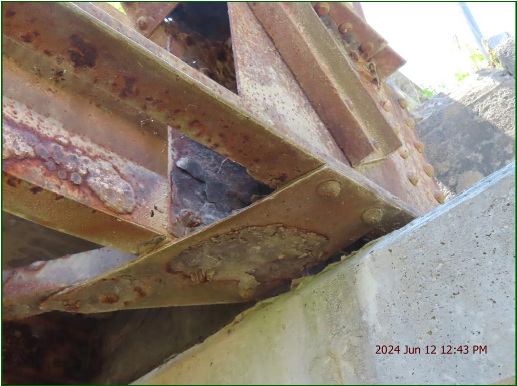
Description: Bottom chord: Medium to severe corrosion at NW with areas of 100% section loss.
