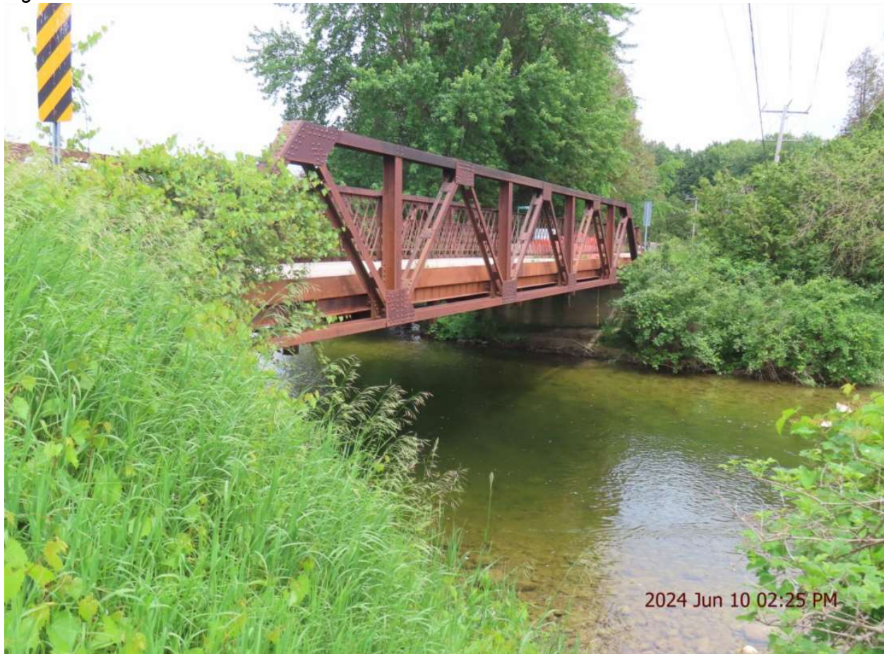
Figure 4.08: South Elevation View of Structure B-020
