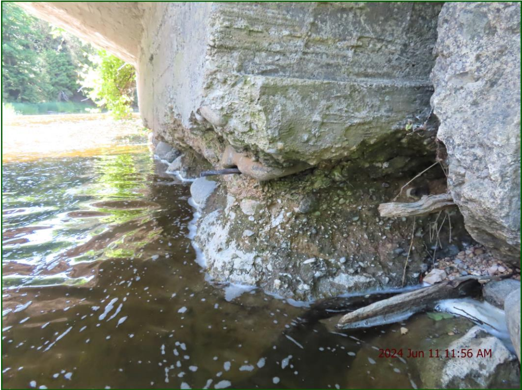
Description: Abutment Walls: Severe scouring and disintegration (2/3).
