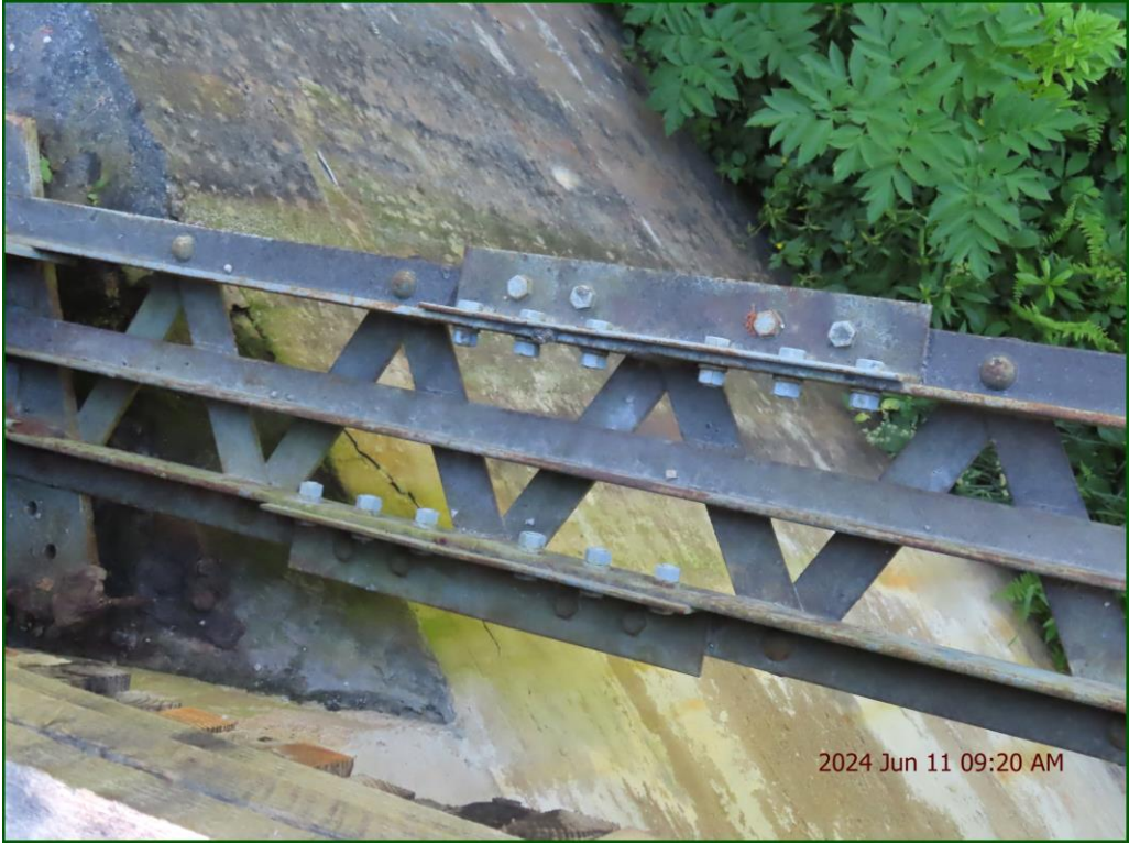
Description: Verticals/diagonals: Railing system welded to structure.
