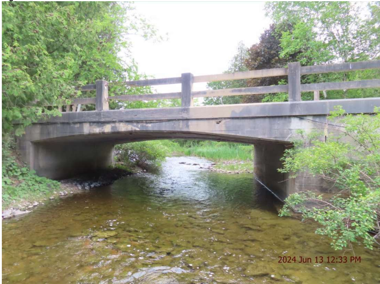
Figure 4.13: West Elevation View of Structure B-008
