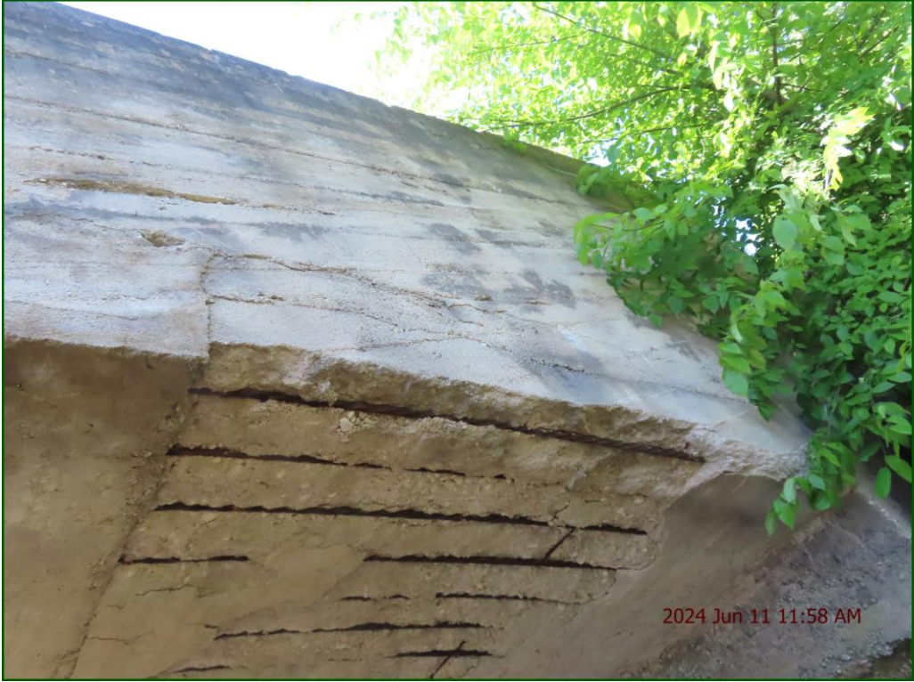
Description: Soffit (ext): Severe spalling with exposed reinforcing throughout (north) (3/3).
