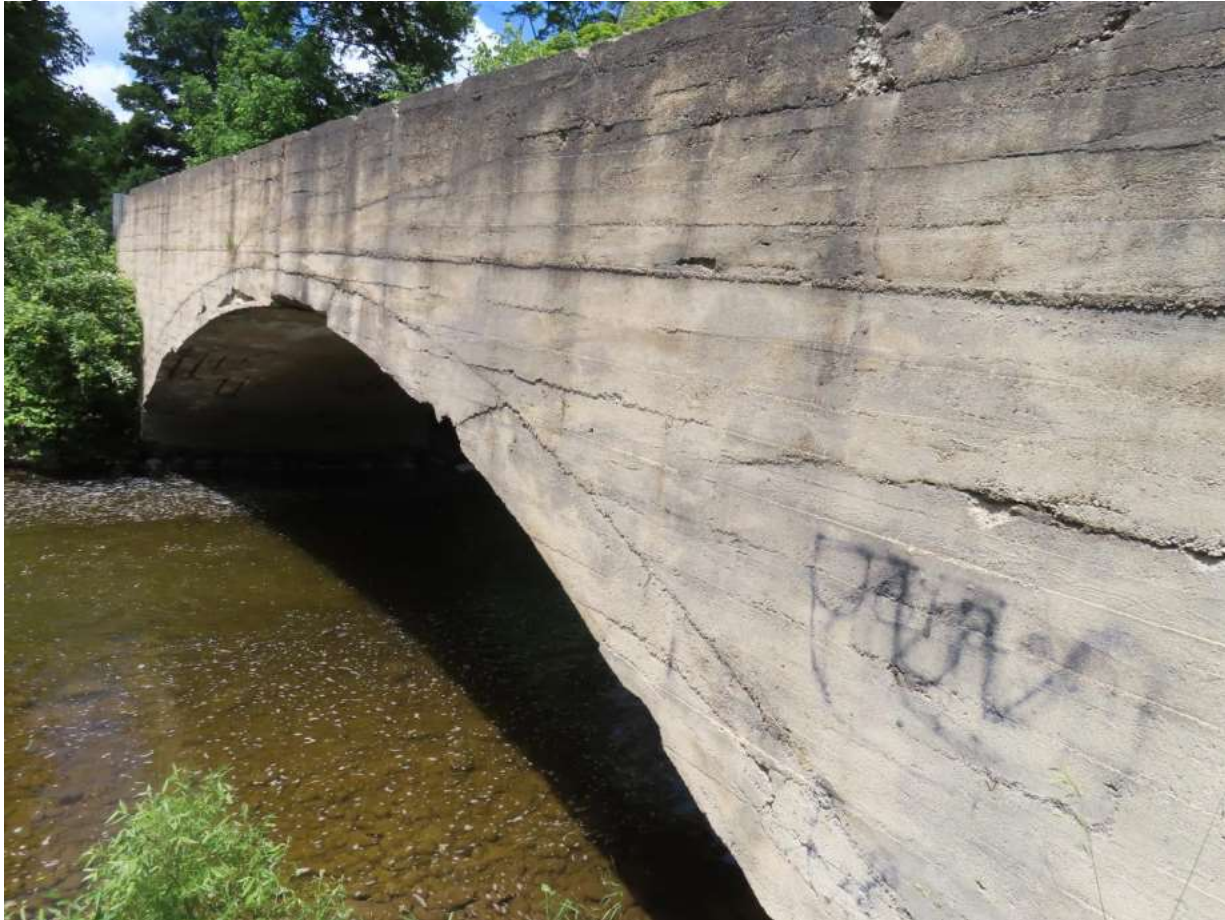
Figure 4.02: North Elevation View of Structure G-038
