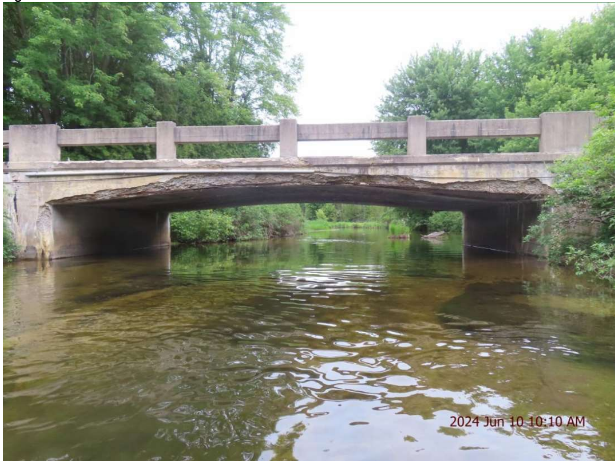
Figure 4.06: South Elevation View of Structure B-003
